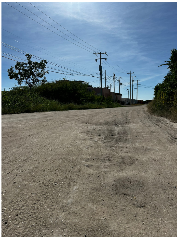
Figure 3.16: Road between Sisal and the campus.
