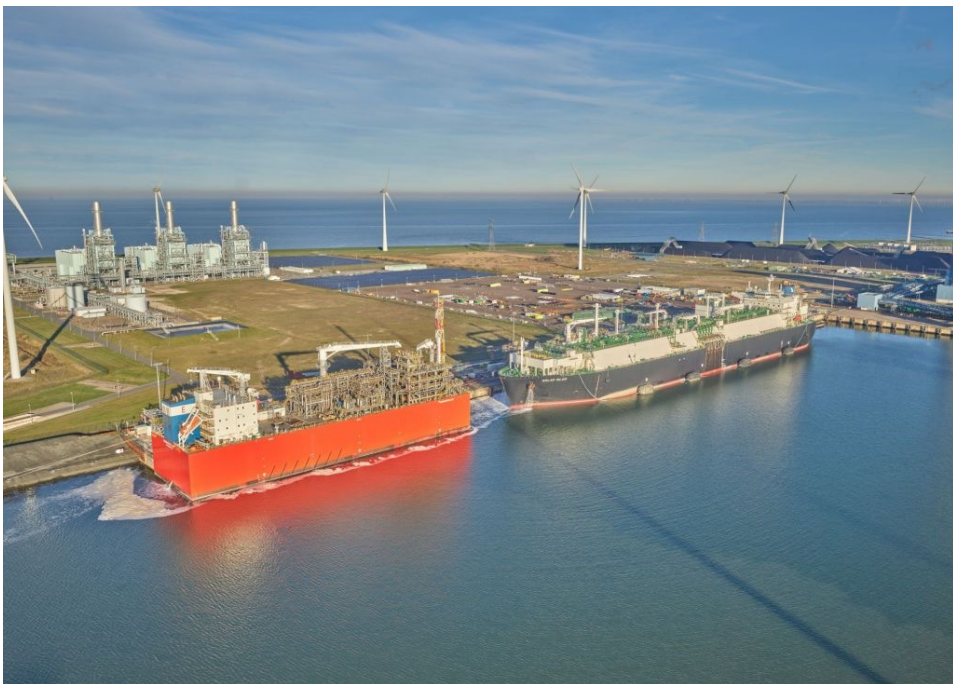
Figure 2.2: EemsEnergy Terminal with 2 FSRUs. EXMAR FSRU on the left [14].
