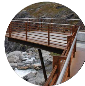
reused steel from demolished INPP buildings
