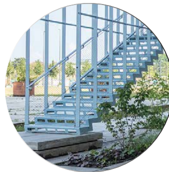
reused steel from demolished INPP buildings
