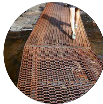
reused steel from demolished INPP buildings
