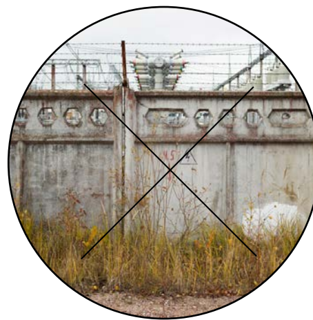
demolition of the fence and reuse it for paving (T2)
