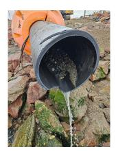
Figure 5.3: Some remaining material in the pipe used to dispose the dredged sediment (De Vincenzi, 2023)
