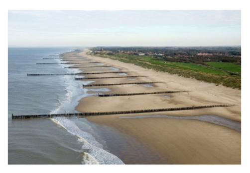
Figure 8.2: Example of permeable pile groynes (Bosboom & Stive, 2023)
