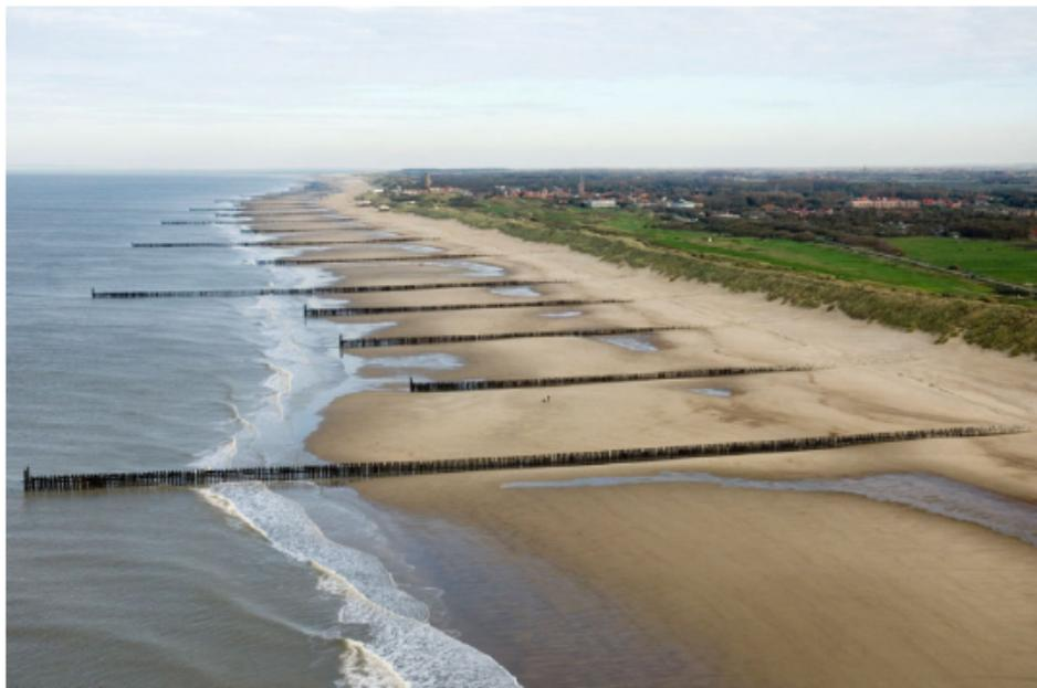
**Figure 8.2:** Example of permeable pile groynes (Bosboom & Stive, 2023)
