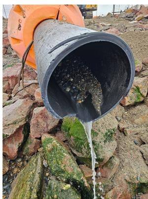
**Figure 5.3:** Some remaining material in the pipe used to dispose the dredged sediment (De Vincenzi, 2023)
