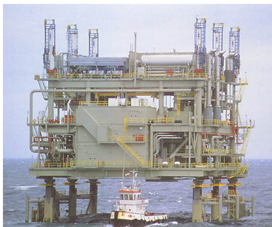
(a) The Epke topsides, the extended legs are visible through the topsides. The hydraulic units are still installed, from Epke.
