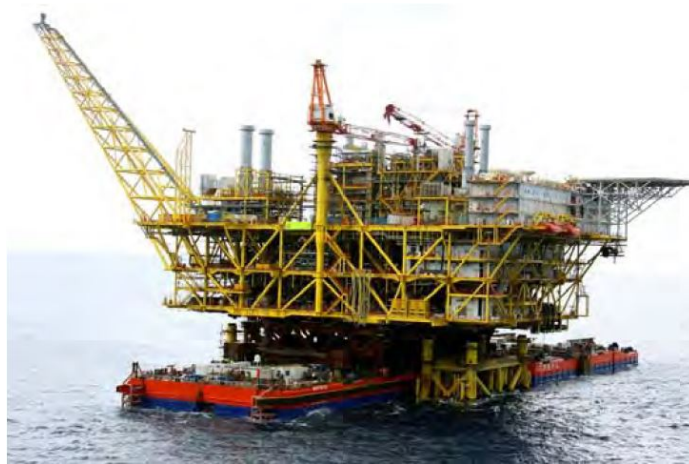
Figure 2.1: The Liwan 3-1 topsides on the HYSY229 barge, just before the mating procedure is started. The heave compensation system will be tested according to this scenario. The main difference is the swell sea which causes more motions of the barge and thus decreases the workability.
