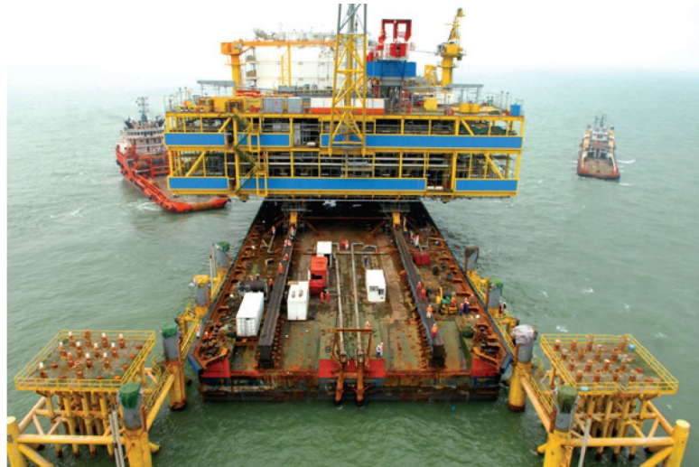
Figure 1.1: Example of a typical floatover operation. The topsides are skidded on a barge, which fits in the substructure slot. The lengthy side of the topsides hangs over the edge of the barge, such that the topsides legs can be lowered onto the previously installed jacket legs, from He et al. (2011) .
