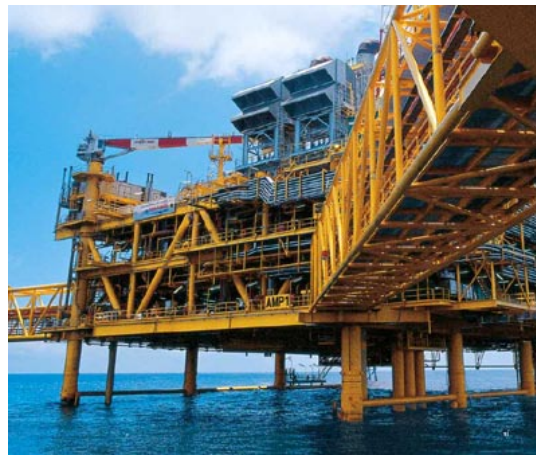
Figure 1.6: The Amenam AMP-1 production platform installed in Nigeria, from (Amenam). The only available information about this project is the installation vessel, the Dockwise Mighty Servant 3. This vessels has a width of forty meters. Looking at the width/air gap ratio it can be estimated that the airgap is smaller than 15 meters.
