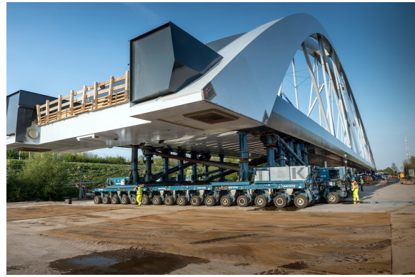
FIGURE 2.8: Railway bridge Muiderberg during movement by SPMTs [Rijkswaterstaat, ndb]
