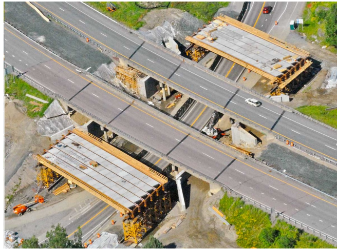
FIGURE 2.4: Lateral slide-in bridge construction [Technical Services, nd]
