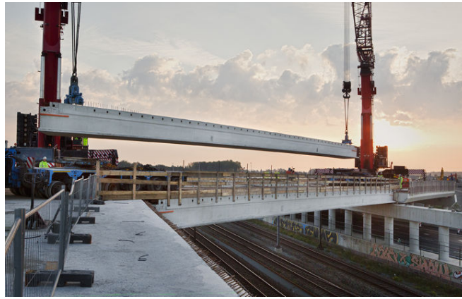
FIGURE 2.2: Erection of prefabricated bridge girders in A9 Badhoevedorp [Spanbeton, nd]
