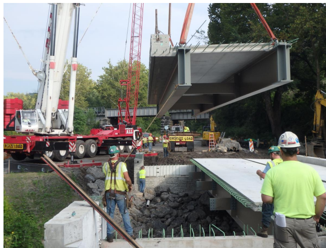
FIGURE 2.3: Prefabricated modular superstructure element placing [Roads and Bridges, nd]
