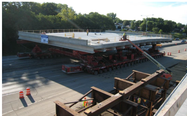
FIGURE 2.5: Superstructure movement by SPMT to the bridge location [Federal Highway Administration, 2015]
