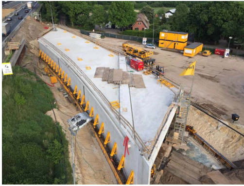
FIGURE 2.7: Lateral slide-in tunnel part in A12 Ede before movement [Heijmans, 2016]
