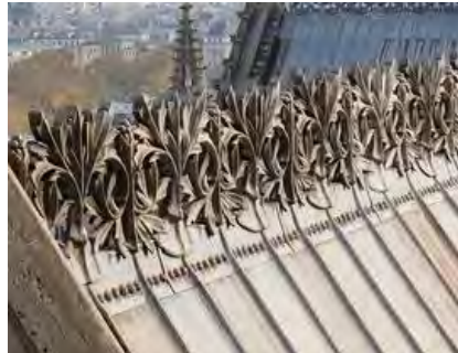
Figure 65 Roof ridge's frieze.
