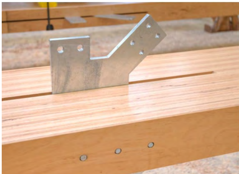
Figure 52 Recessed steel plate connection in Baubuche (Pollmeier, 2020).
