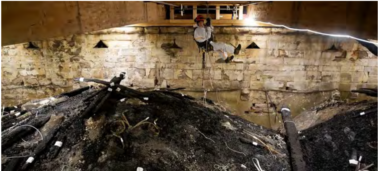
Figure 34 Hanging workers from the ceiling, hovering above the labeled debris (Zachmann, 2020).
