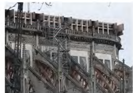
temporary cassettes on top of clerestory wall
