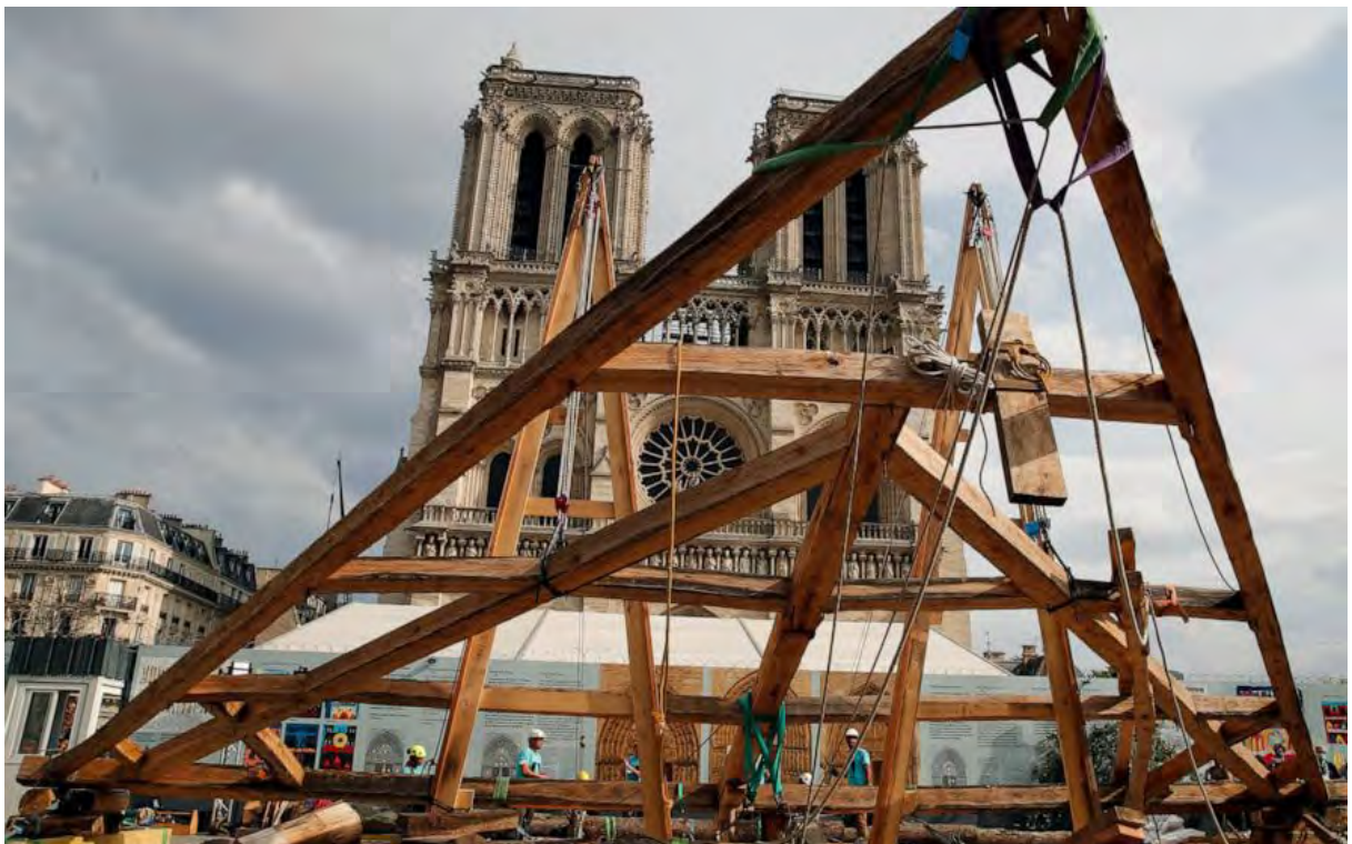
Figure 85 Contrasting manufacturing and assembly strategies are adopted by the authorities. Top: modern timber structure to stabilize vaults. Bottom: medieval techniques utilized to reconstruct example truss (Zachmann, 2020).
