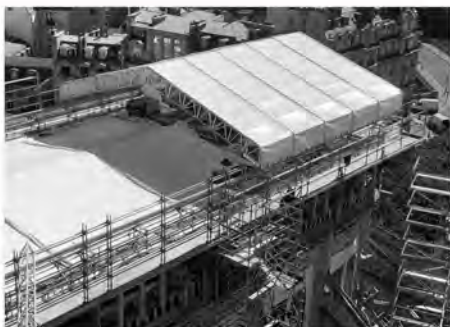
temporary aluminium roof on top of glulam structure
