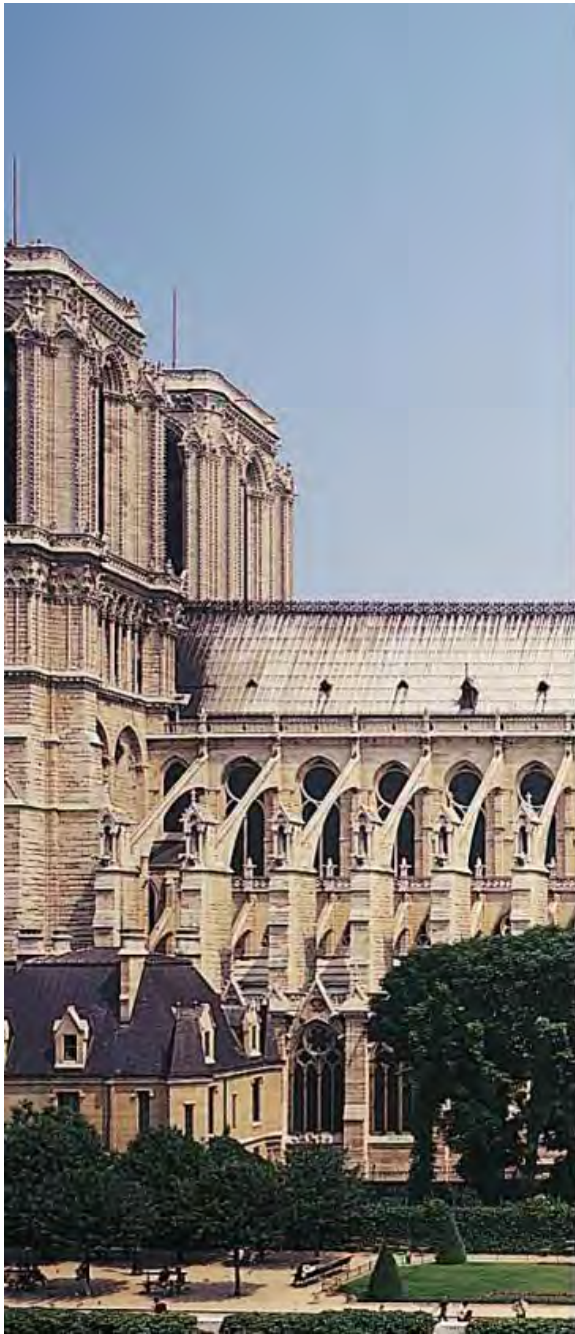
Figure 26 Notre Dame de Paris seen from the south. The transept is taken away to reveal the different systems of flying buttresses of the choir and the nave (Notre Dame de Paris, 2003).
