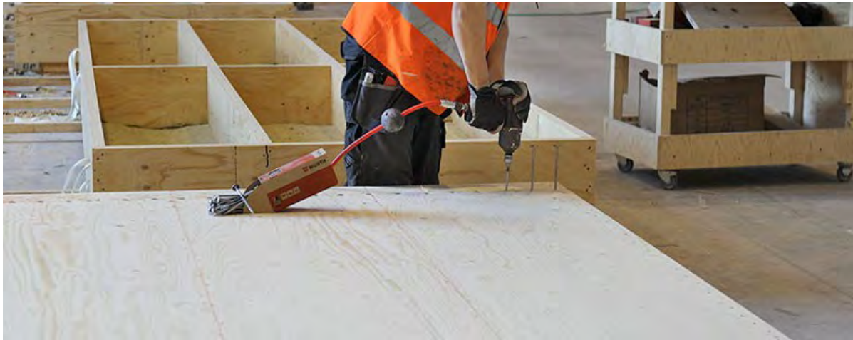
Figure 49 Production of prefabricated LVL cassettes (Stora Enso, 2016).
