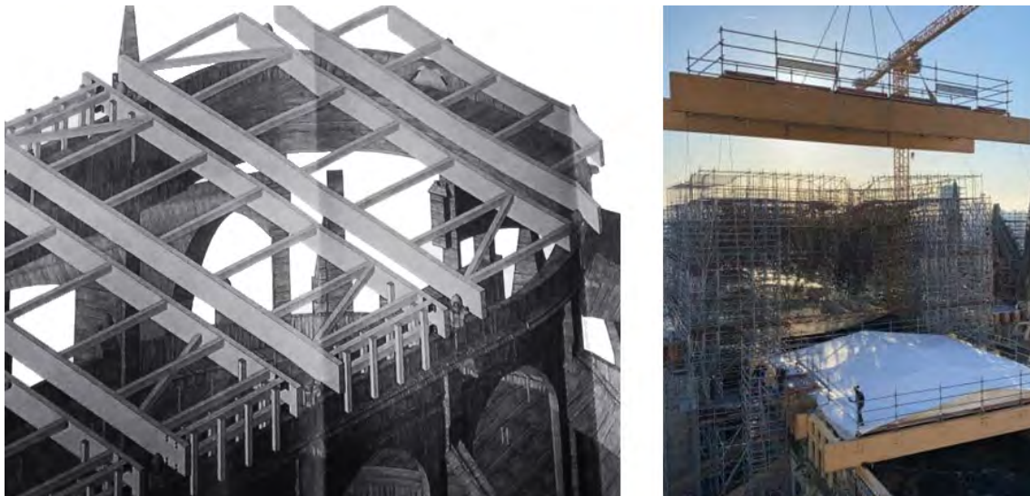
Figure 32 Left: Overview of prefabricated Glulam cassettes positioned on top of the guttering wall of the choir. Right: photo showing moment of placement of cassette (Zachmann, 2020).
