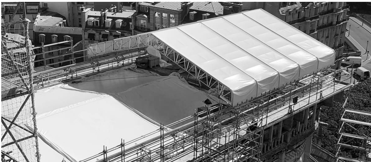
Figure 35 Temporary tent to protect construction workers and debris from rain and sun (Zachmann, 2020).
