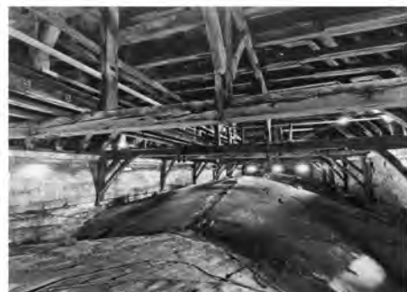
former timber roof structure: The Forest
