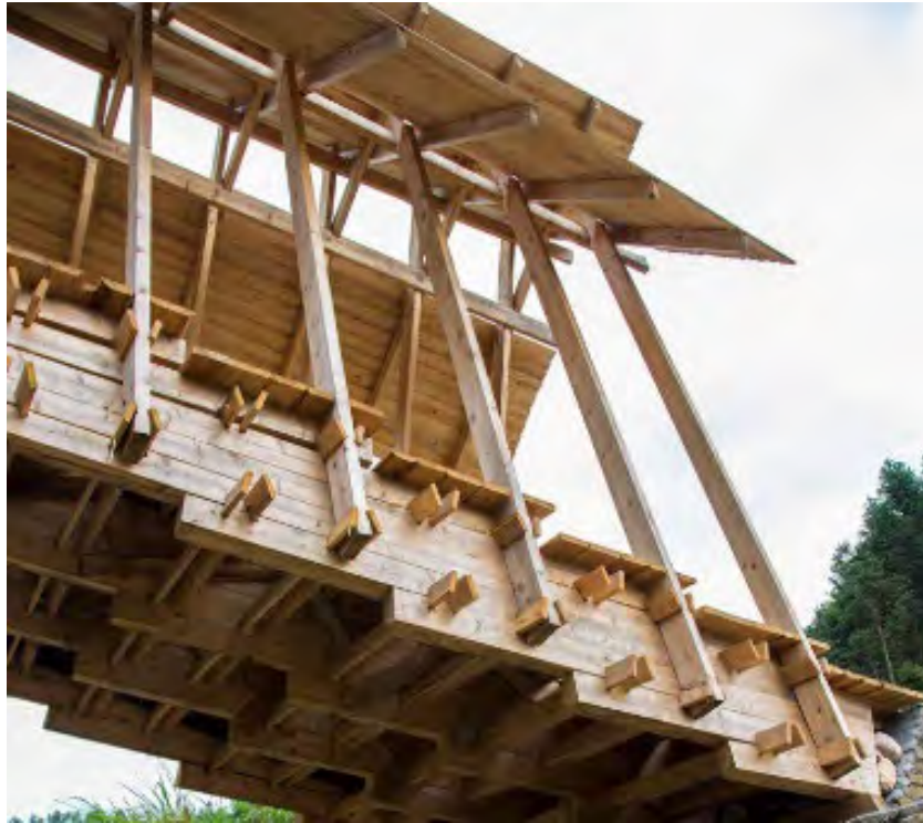
Figure 51 Wind and Rain Bridge, connections without any mechanical fasteners (Holohan, 2018).
