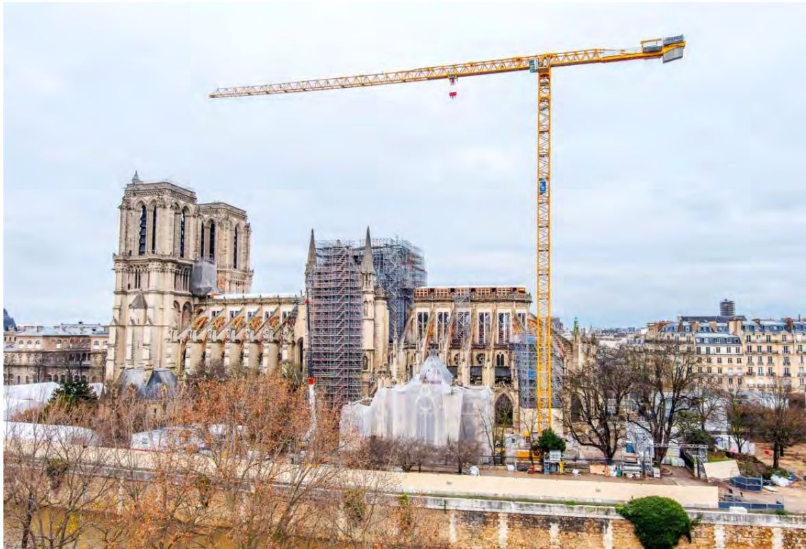
Figure 37 Potain MDT 809 Tower Crane at Notre Dame de Paris (Zachmann, 2020)
