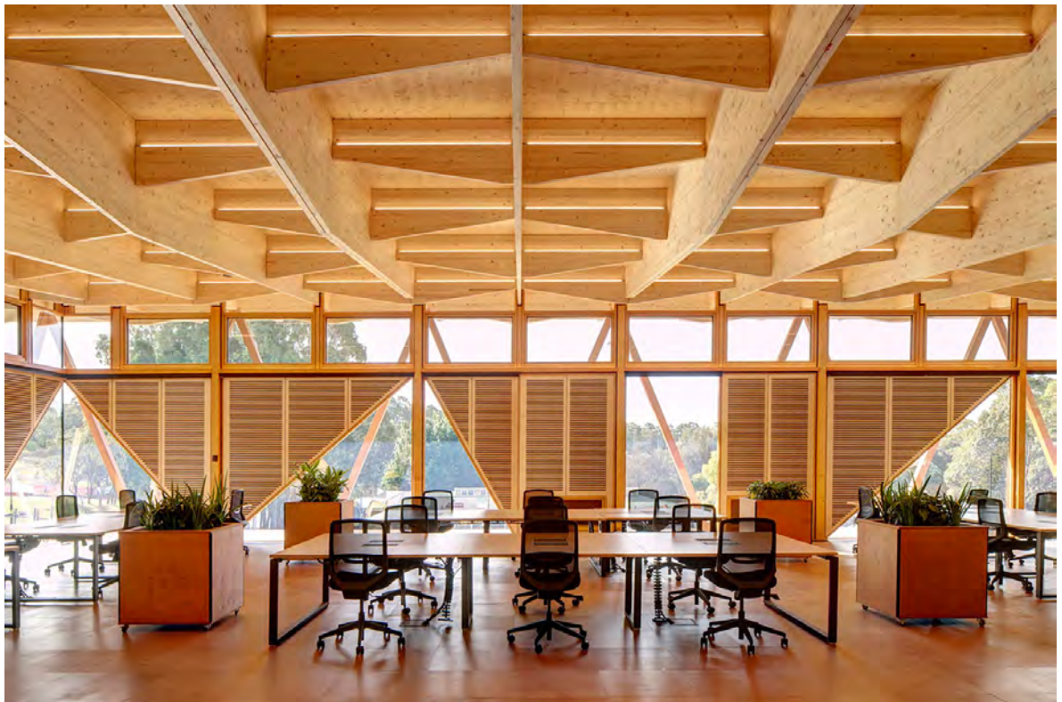
Figure 48 Macquarie University clearly showing the doubling of the primary beams (Arup, 2018).
