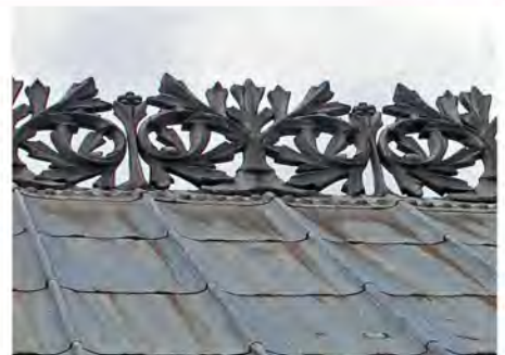
new (old) roof timber roof structure and cladding
