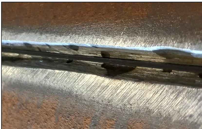
Figure 4.6: Fibre optic cable within the prepared groove of the SIc pile
