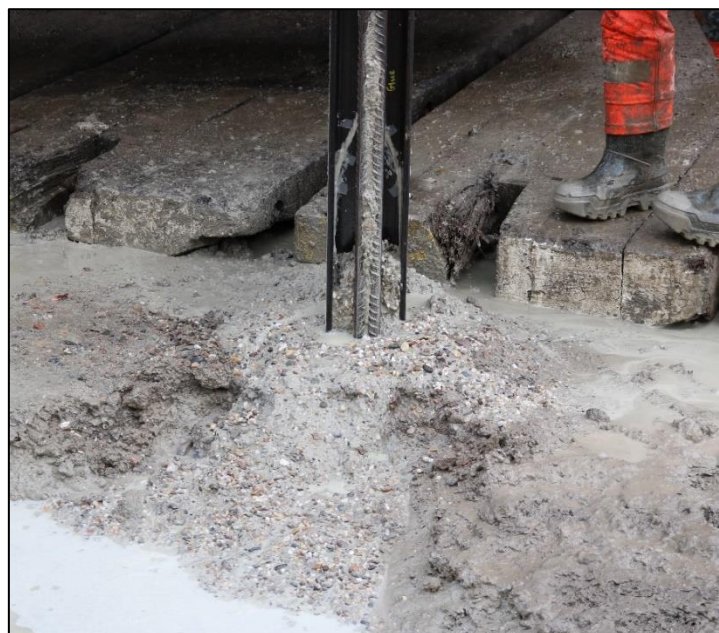
Figure 3.6: Pile F2 following installation, showing the coarse aggregates surrounding the pile
