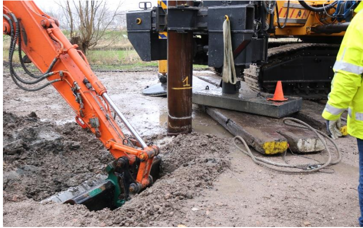
Figure 3.8: Trench in front of pile to collect outflowing grout
