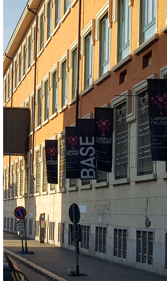
Signage flags exposed on the facade of the Event Centre
