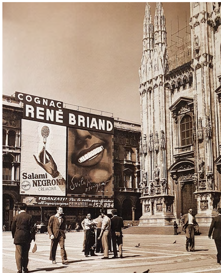
Piazza Duomo 1973 The Facade of buildings are used to install advertisement Billboards
