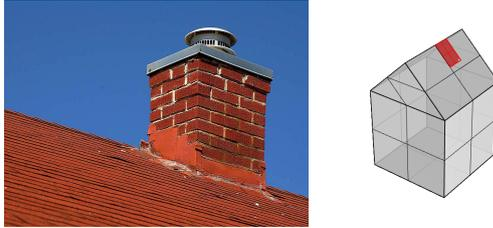
Figure 1.13: Instead of modeling the chimney (left, source: wikimedia) as such it can also simply be indicated semantically in an existing LOD2 model (right, nb: assuming the chimney size is below the custom threshold to include it in LOD2).
