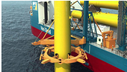
Figure 3.6: Example Fixed monopile gripper frame [17]
