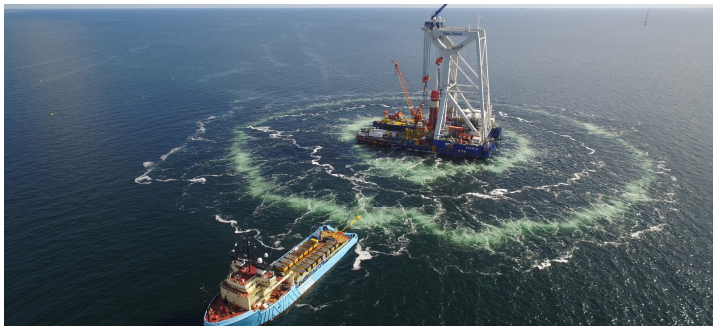
Figure 1.8: Mono-pile installation with the Svanen, [Van Oord, 2017]
