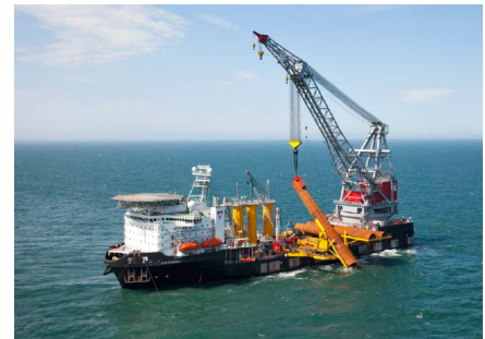
Figure 1.9: Mono-pile installation with the Oleg Strashnov, [heavyliftnews, 2016]
