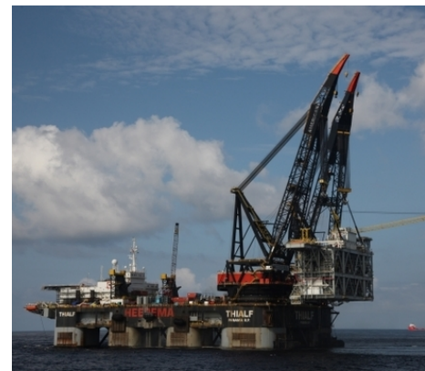
Figure 1.12: Crane operation (HMC)
