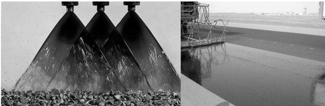
Figure 2-1 Bitumen emulsion is sprayed onto the pavement for surface dressing
