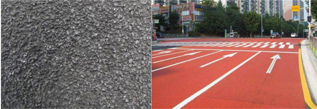
Figure 2-3 Antiskid surfacing on runways (left) and colored antiskid surfacing at a traffic light area (right)
