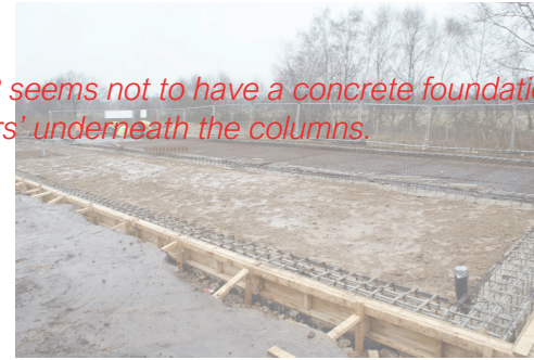
Pouring of the foundation and the floor
