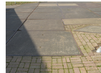
C Fig: brick pavement “basketweave”
