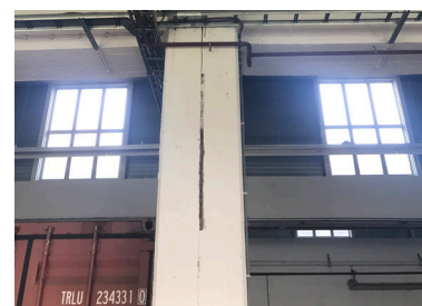
Fig: Shell roof windows
