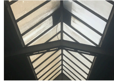
Fig: Steel roof window frame
