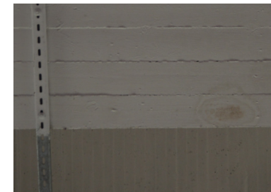
Fig: Concrete beam with wood casting
