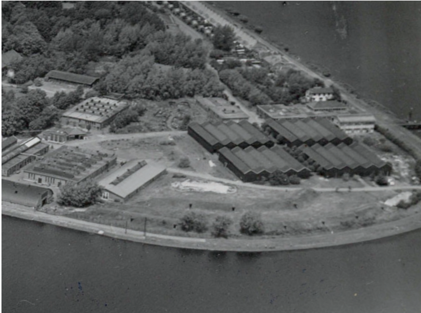
Green Head of the Cape with: Peat sheds, shelters, building 421 (the Wash House) Date unknown: approximately around 1941
