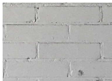
Fig: White painted bricks wall
