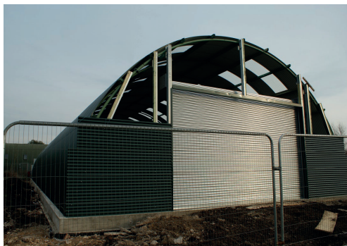
Finishing the side facades
