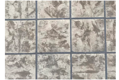
Fig: Square brick floor
