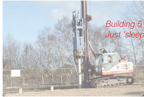
Pile driving for the foundations
