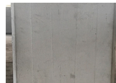
Fig: Concrete column with wood casting
