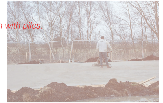
Smoothing the concrete base.
