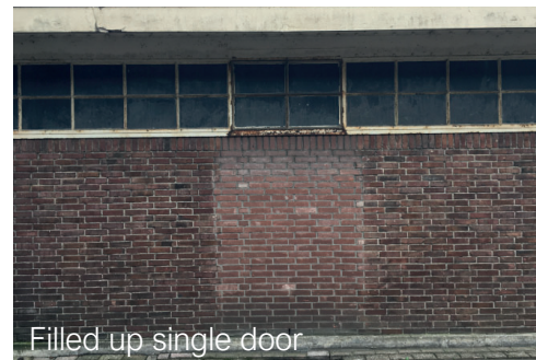
Filled up single door and new doors
