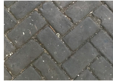
Fig: Single herringbone brick floor
