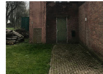
B Fig: brick pavement “diagonal herringbone”
