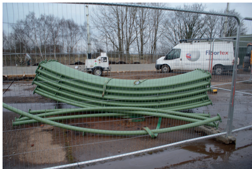
Assembling the main steel trusses
