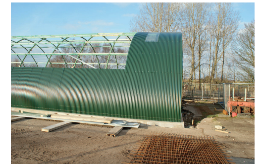
Adding the exterior facade (steel plates)
