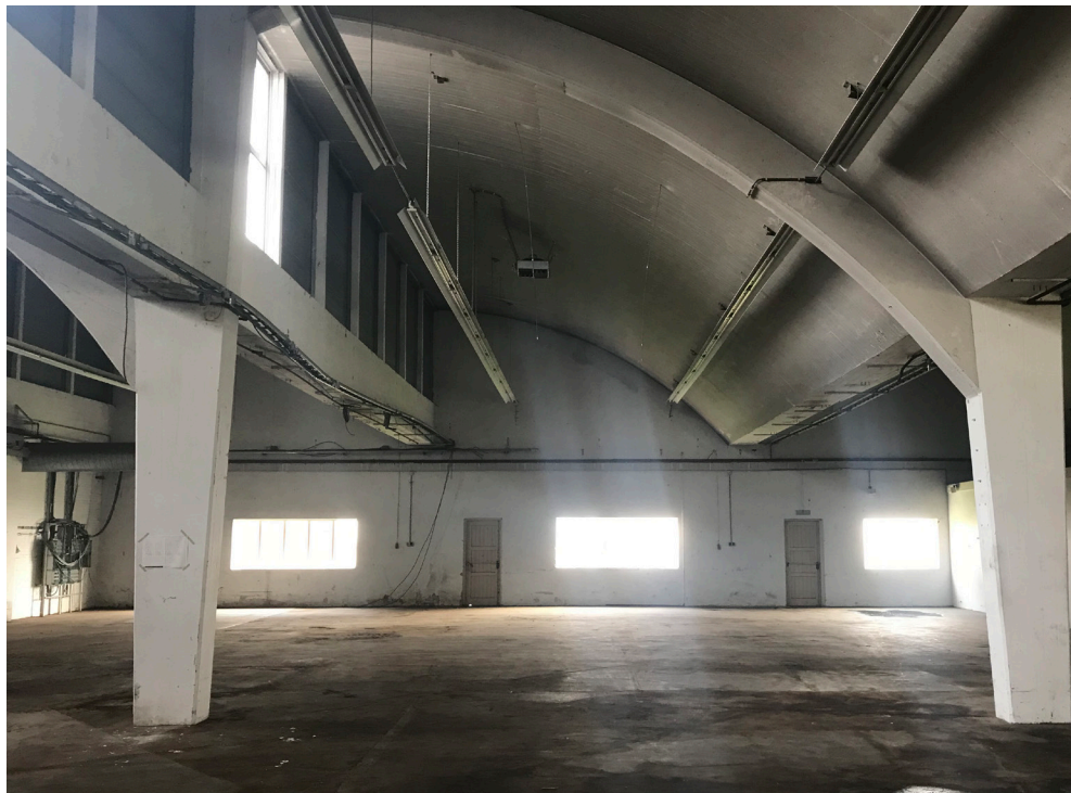
Fig: Concrete shell roof with wood casting
