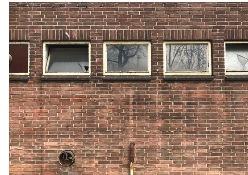
Fig: Small window for toilet
