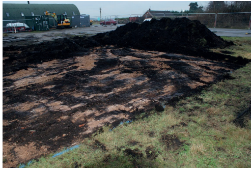
Preparing the ground
