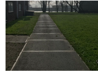
A Fig: concrete pavement
