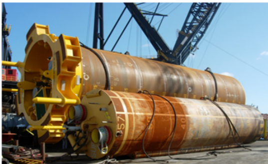
(a) Suction piles, with valves on the top plate
