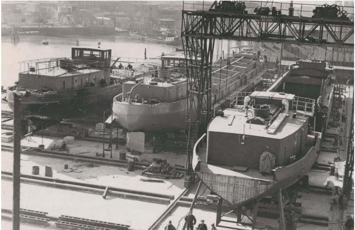
Figure 21 A photograph from 1948 shows the new “Amerikaanse Helling,” on which French ships were assembled in series. The ships progressed step by step towards the Wantij, where they were finally lowered into the river when finished (Van ‘t Verlaat, 2017) (Source: RegionaalArchiefDordrecht, n.d.).
