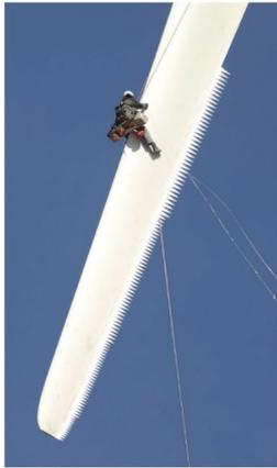
(a) Serrated wind turbine blade
