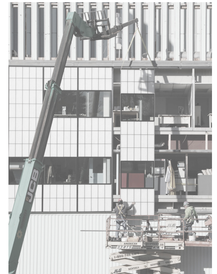
Kalwall facade system. 1. Kalwall Weatherable Coating (KWS) 2. The Bond Line 3. Exterior Fiber-Reinforced Polymer (FRP) face sheet 4. Translucent Insulation (TI) Lumira aerogel. 5. Interior Fiber-Reinforced Polymer (FRP) face sheet 6. Structural Grid Core composed of a series of interlocking aluminum and thermally broken I-beams. Source: https://www.kalwall.com/resources/?resource_type=cad-details
