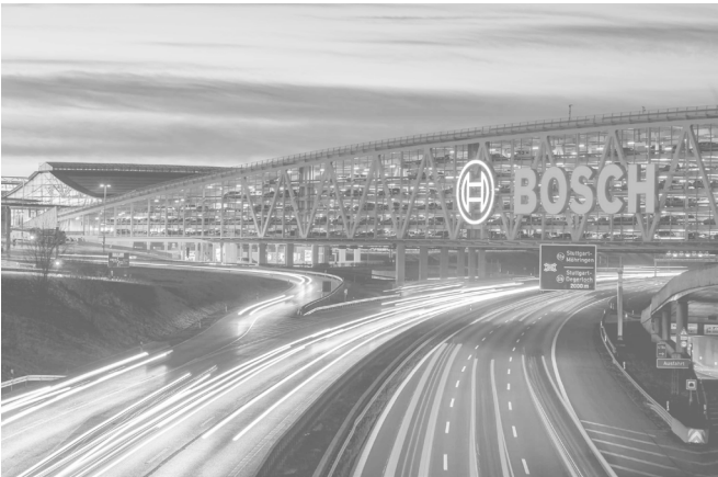
The Bosch Parkhaus building above the motorway in Stuttgart. (Spans range from 85 to 105 metres). Source: https://www.btc-echo.de/wp-content/uploads/2023/02/shutterstock_1814136131-scaled.jpg
