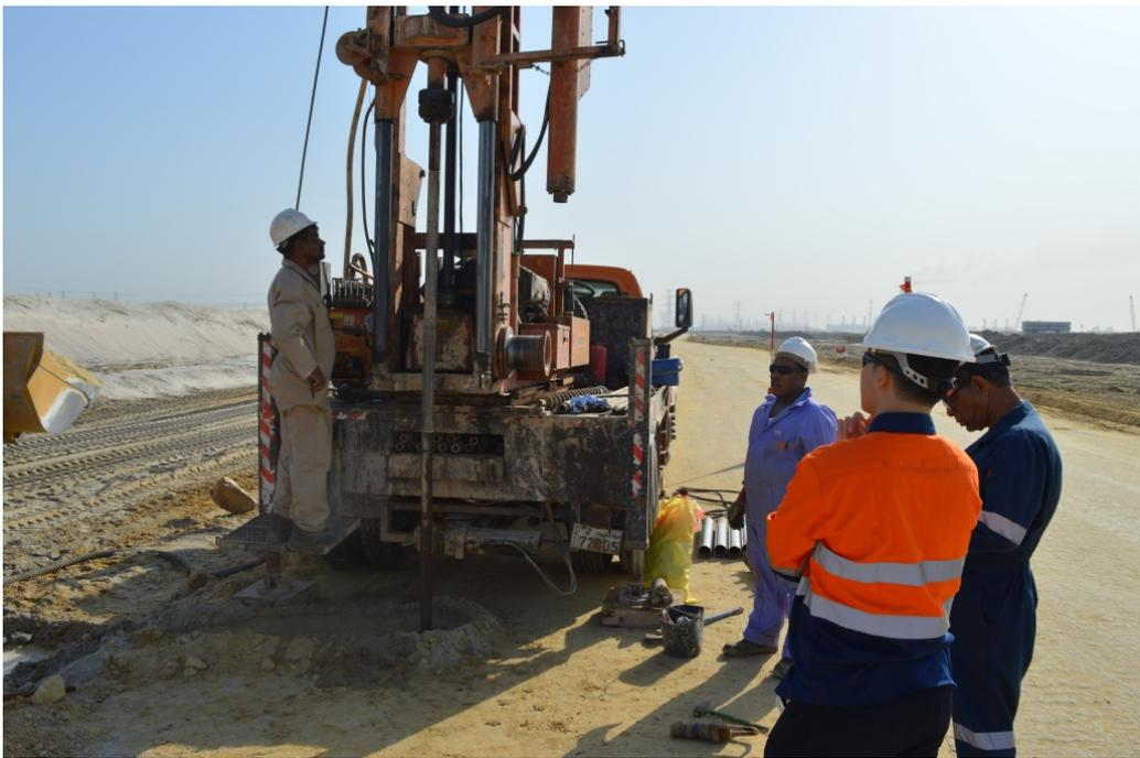
Figure F.3: A boring being executed.
