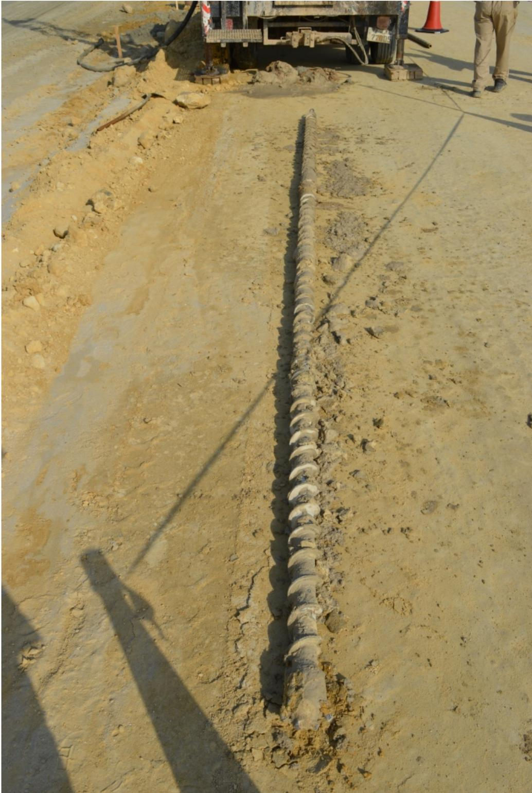
Figure F.5: An 'exploratory' boring, a quick and dirty method.
