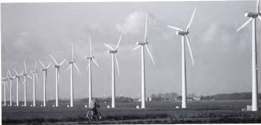
FIGURE 2.4: An example of wind turbines placed on farmer land property. Consisting of 19 Micon 600 kW turbines, in 1999 was the largest installation, exploited by a cooperation of six windboers (IEA, 1999)
