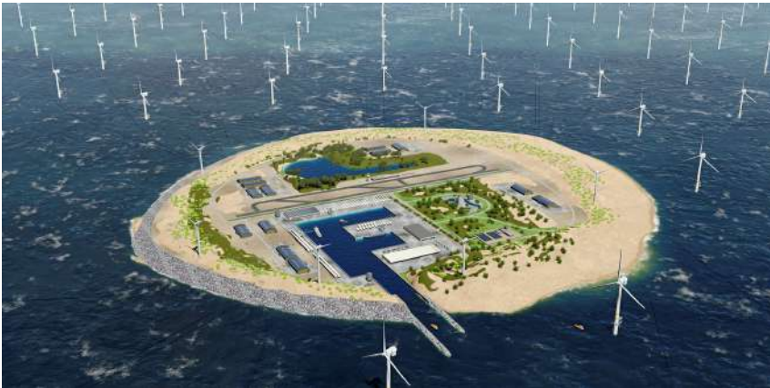
FIGURE 2.7: Digital representation of the concept of the North Sea Energy Hub in the Dogger Bank, implementing wind, power-to-gas and power-to-hydrogen technologies. (TenneT, 2020)
