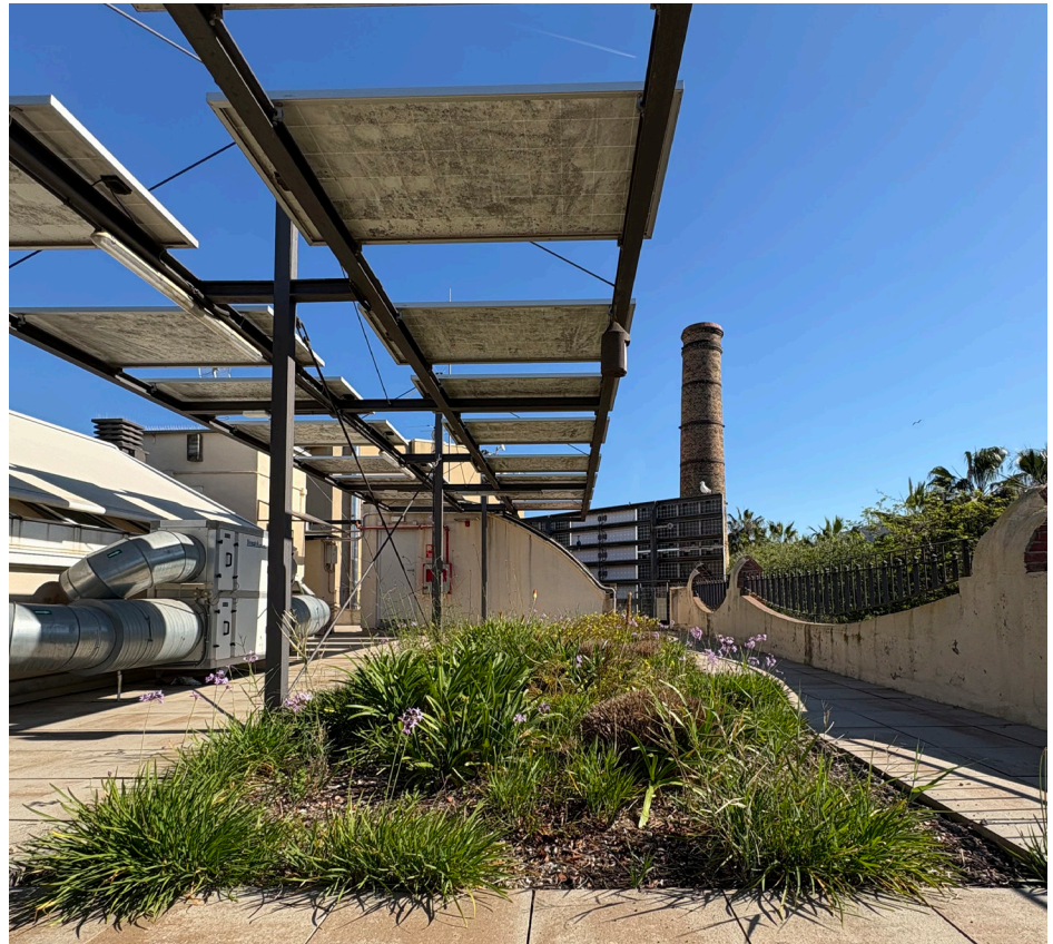
Blue & Green Roof
