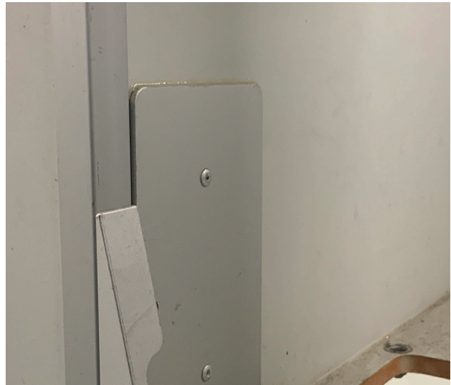
Fig 3.6. Revets with bonded bracket
