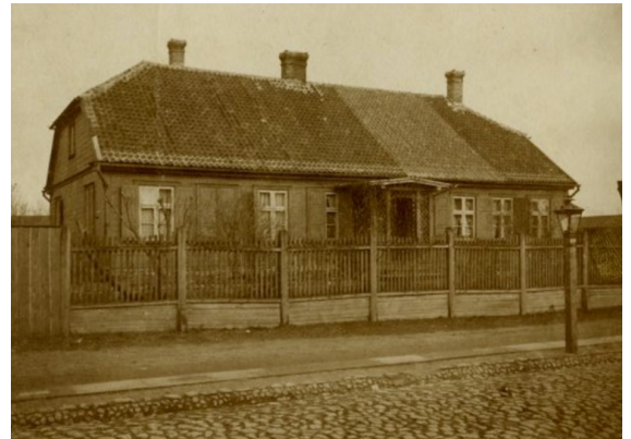
Fig. 23 Riga. An old residential building at 237 Maskavas Street (1900)
