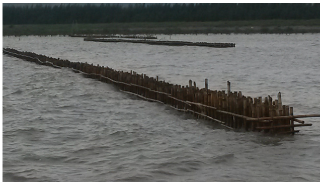
Figure 3. Bamboos with reed filling in the gaps being used as wave screens along a T-groyne in Vietnam (photo by H. J. Verhagen)
