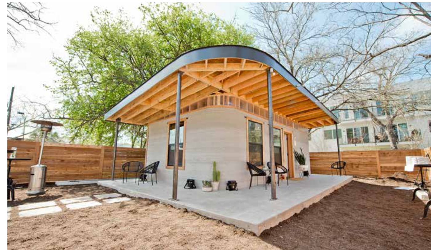
Housing unit printed in 24 hours
