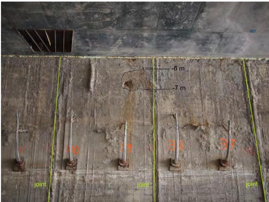
Figure 28: Location of the sand inclusion in the Delft field case relative to the joints and panels
