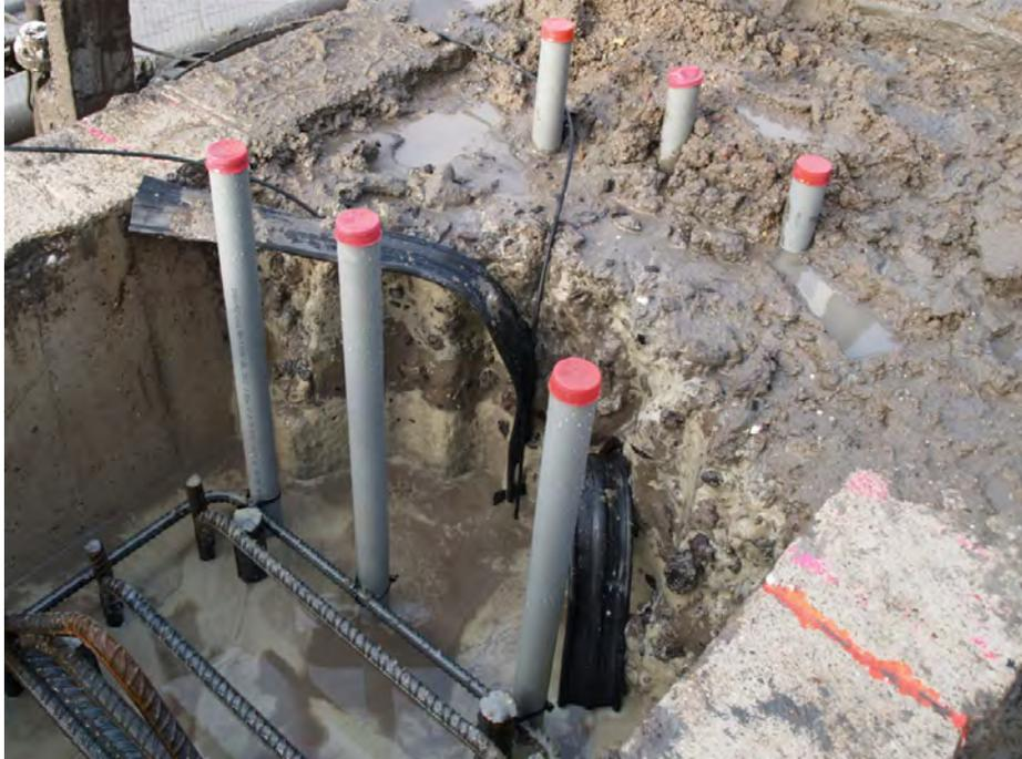
*Figure 7: Joint between a cast panel and an excavated panel, just before concrete casting (showing a total of 6 CSL tubes)*
