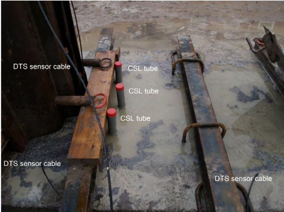
Figure 6: Panel after concrete casting, showing the CSL tubes and the DTS sensors
