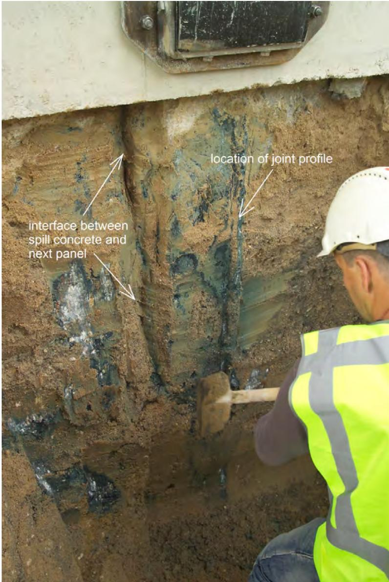
*Figure 77: Picture showing the intended joint and the accidental extra joint due to non-removed spill concrete*
