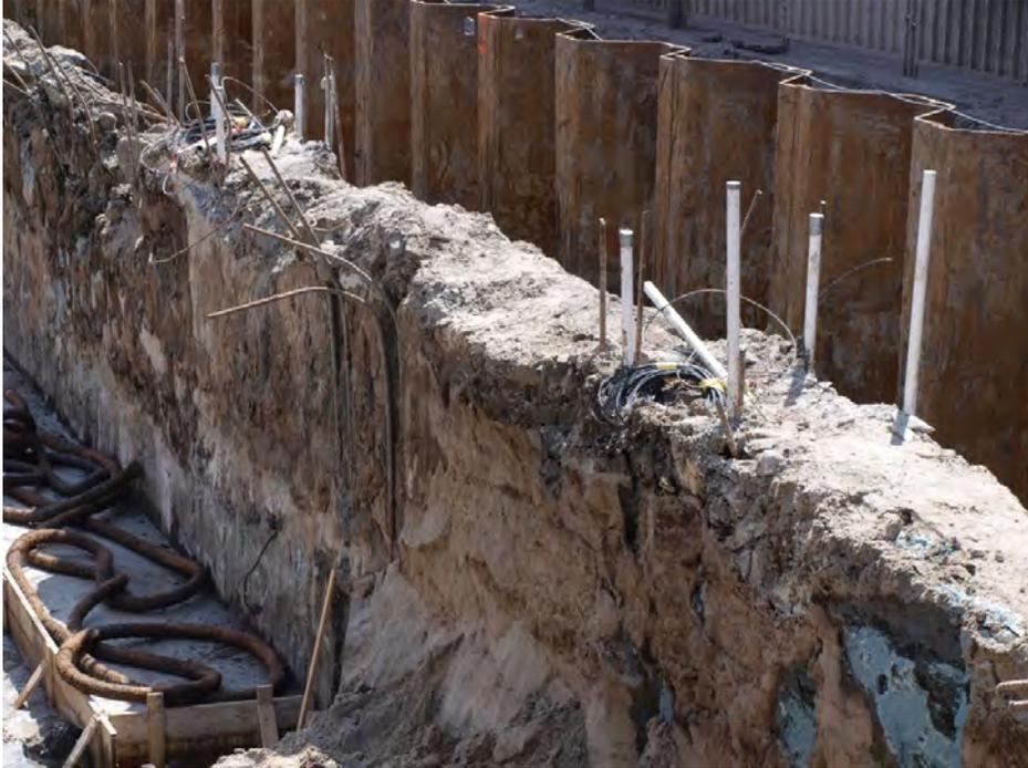
*Figure 4: Top of diaphragm wall just before demolishing top meters, note the CSL tubes*
