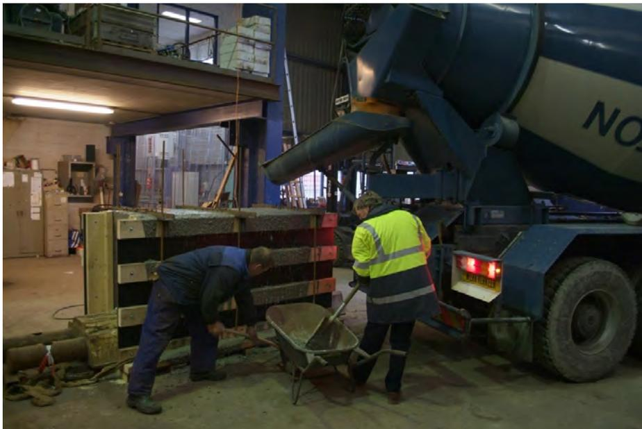
*Figure 2: Test block casting*
