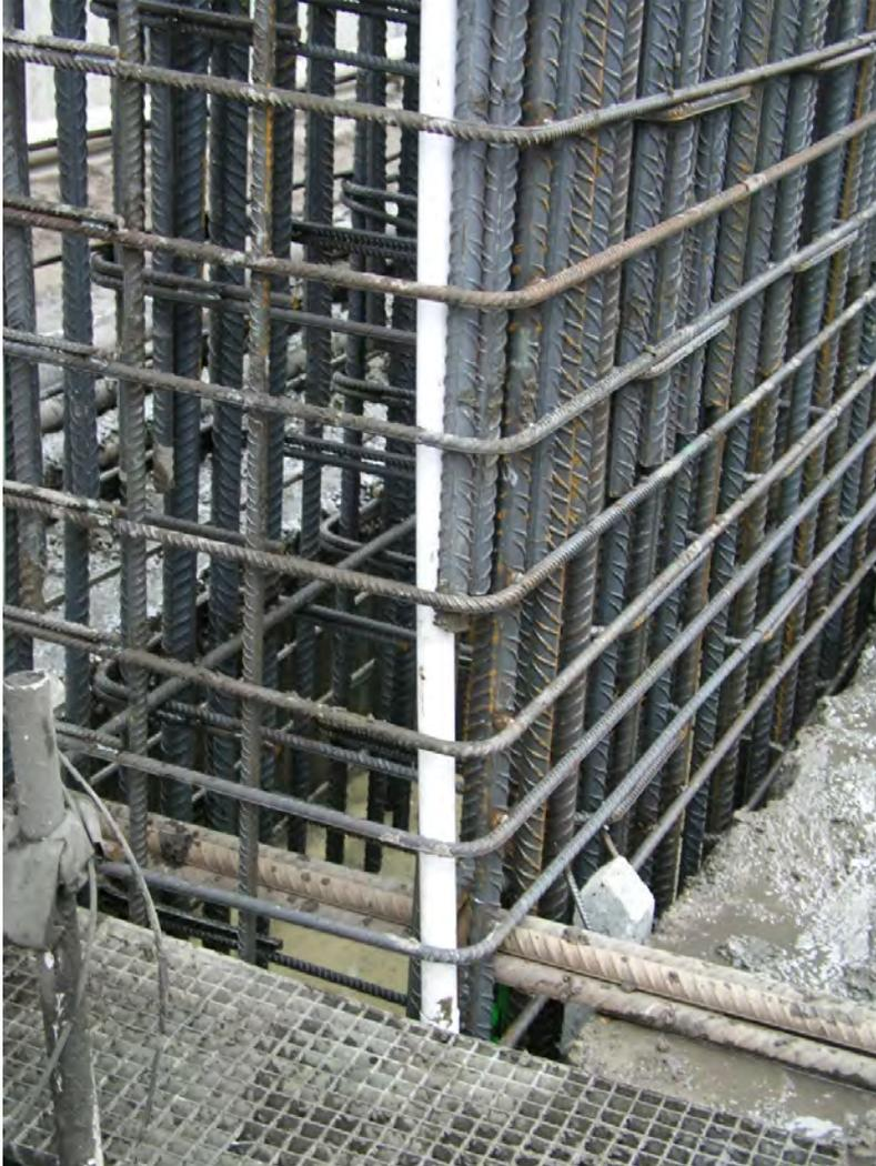
*Figure 5: Rebar cage with PVC tubes at connecting height of two sections*
