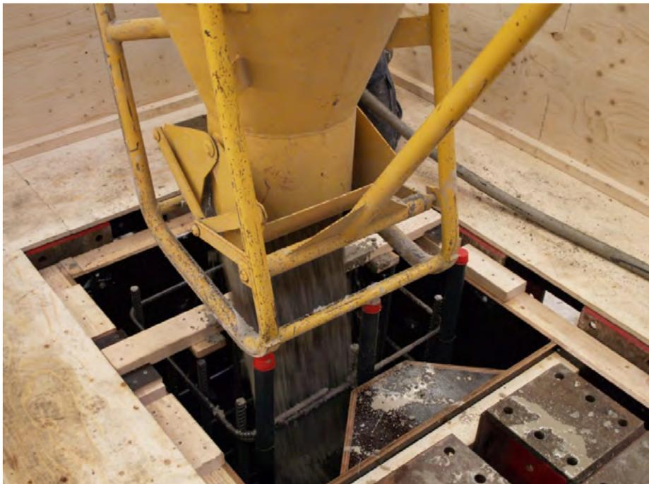
*Figure 9: Concrete casting of the one of the test objects*
