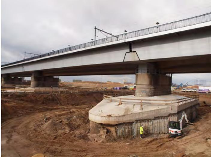
*Figure 78: Temporary situation before diaphragm walls are covered with high quality concrete cover*
