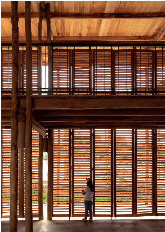
three references of openable facades, where the woven bamboo or wooden louvers allow flexibility for both use and interpretation.
