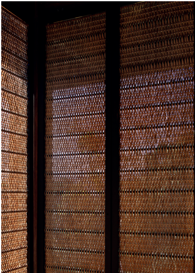
three references of openable facades, where the woven bamboo or wooden louvers allow flexibility for both use and interpretation.
