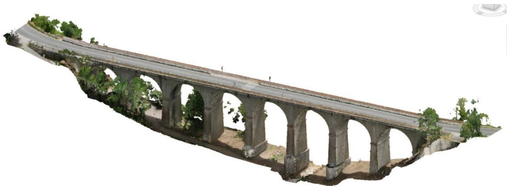
Fig.2 Point clouds of the inspected infrastructure
