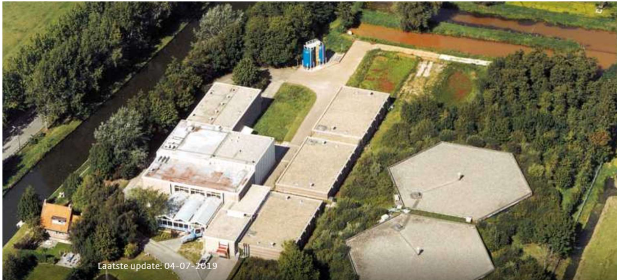
Figure 3-13 Kamerik treatment station.
