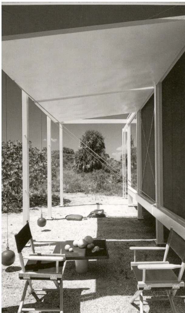
Exterior view of the pulley system in opened position, creating outdoor living space.
