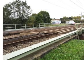
(c) Transition zone side view (from ballast to slab track)
