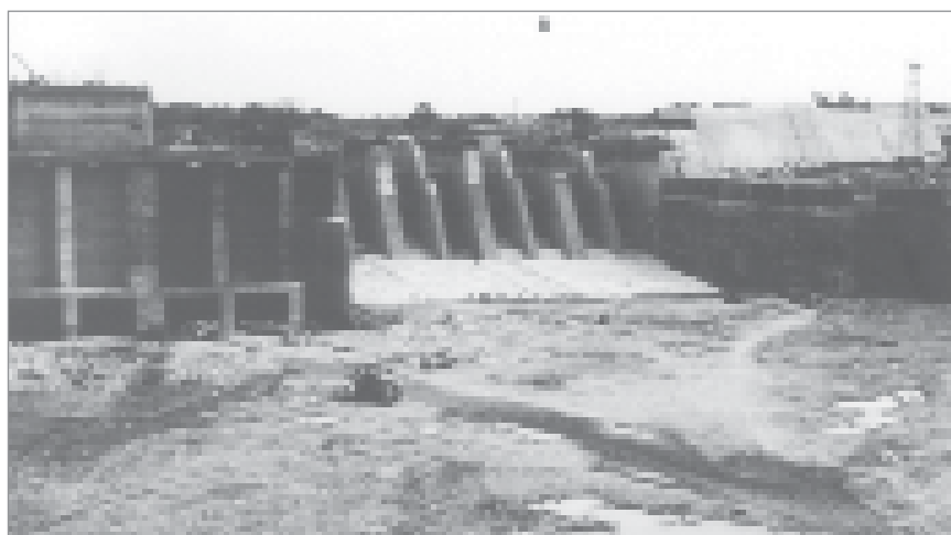
Figure 7.17 Diversion stage II of the River Niger at Kainji Dam will take place through unfinished spillway structures (courtesy J van Duivendijk)
