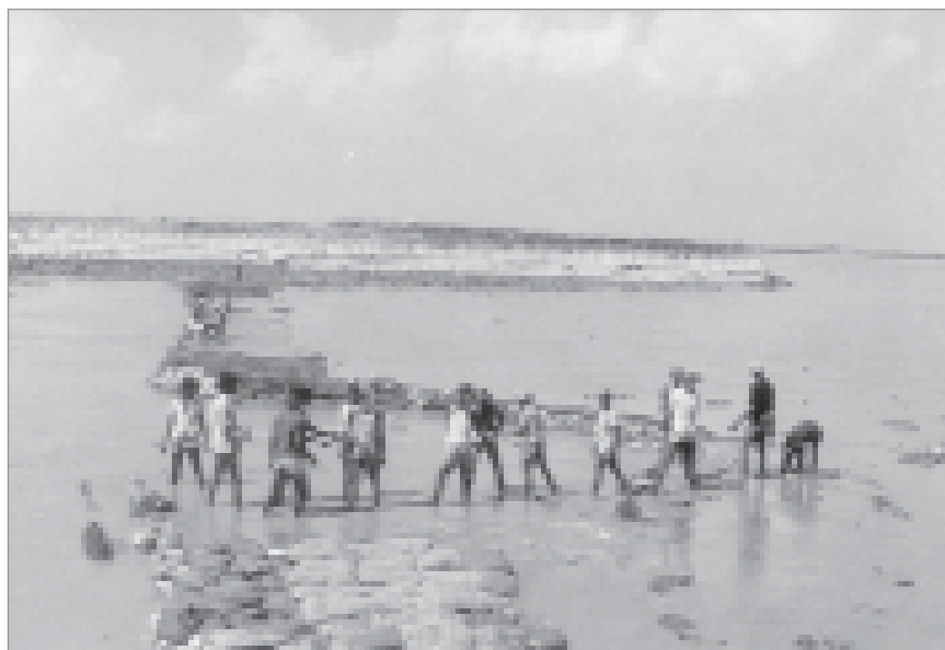
Figure 7.29 Sill in estuary closure, Feni River, Bangladesh (courtesy J van Duivendijk)
