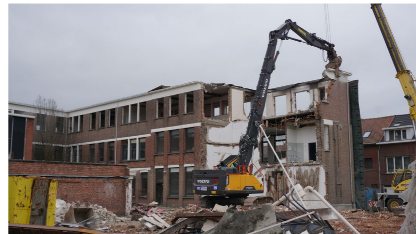
The machine is eating from the building. 'Knippen' they called it, since it needs to cut through the reinforcement of the concrete. A process that's way harder than demounting the bricks, where they let part of the wall fall and it breaks in several pieces, removed by the handlangers.
