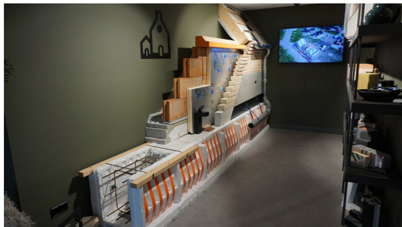
A 1:1 facade detail showing the layers of the facade. Some interesting insights can be derived from this. All visible elements are fitting in the philosophy that the Kempische bouwstijl consists of natural and reused materials. However, practically everything that is not visible is not in line with that philosophy. It shows how KempIQ is treating reuse in the most cost efficient way possible, not using any reused material too much and covering which doesn't match the desired patina. The photo below shows reused bricks on top of new ones.
