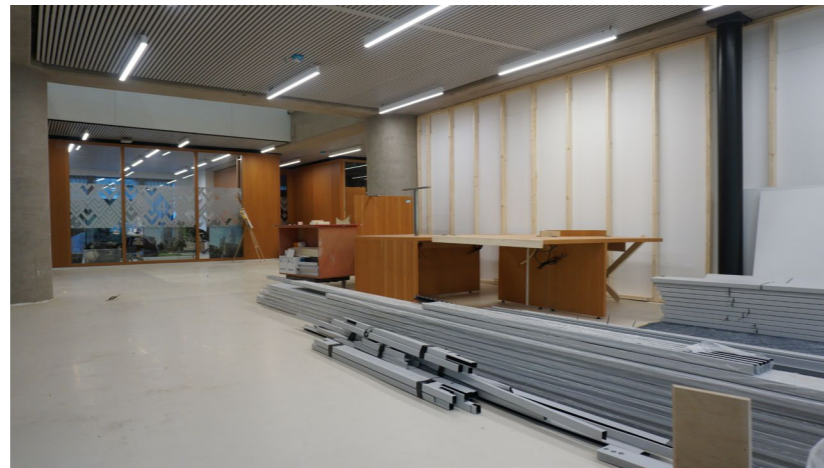
One of the partition walls we removed, mainly consisting of MDF pieces, wrapped by a layer of finishing.
