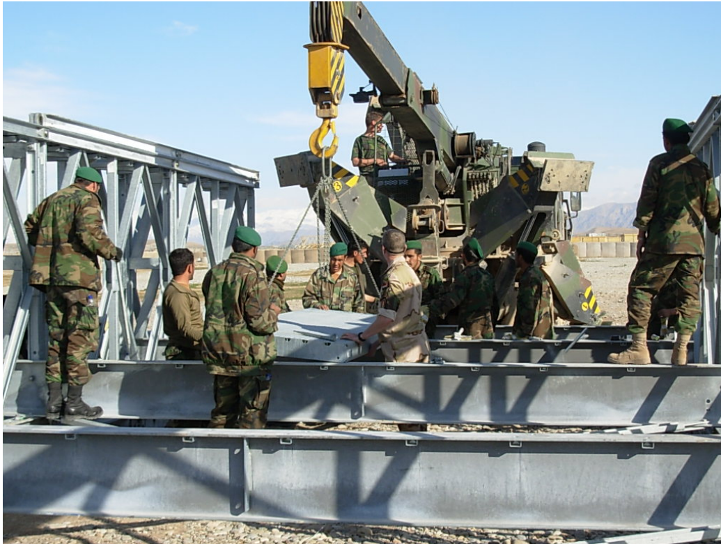
An impression of the ANA engineer training. Here the engineers were taught how to construct a Mabey and Johnson bridge.
