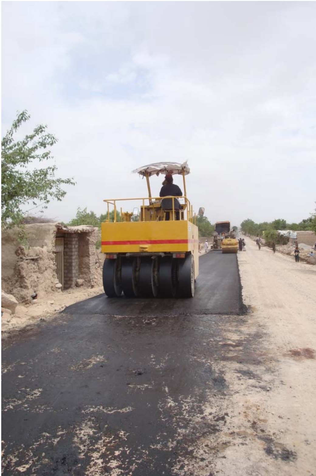
An asphalt roller in action. This road section was located close to a populated area.
