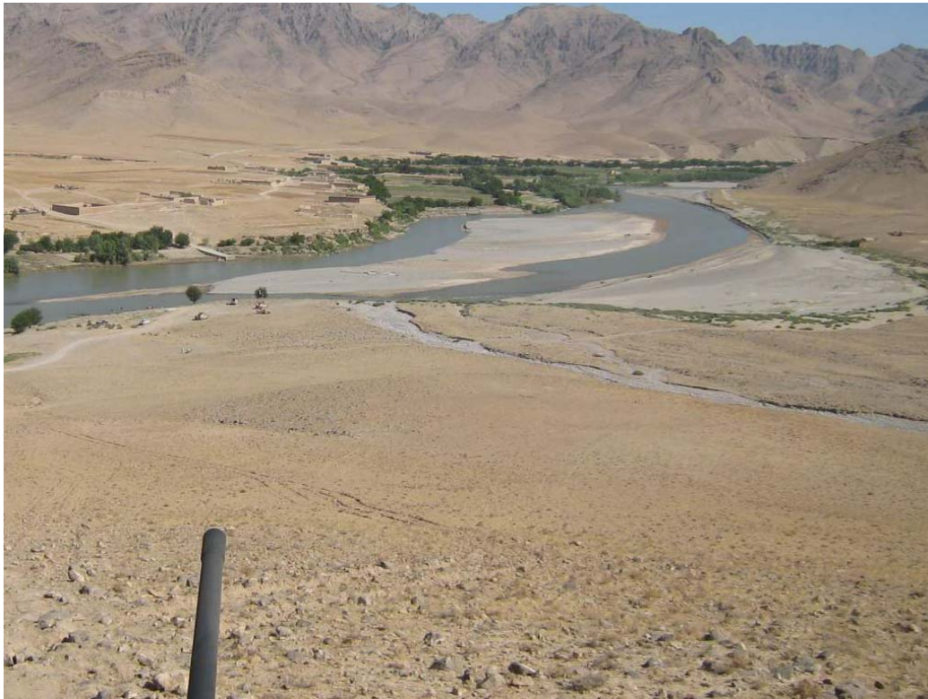
This picture was taken from the hill on the east side of the embankment showing the crossing after the spring flood. On the middle sand bank in this picture the east abutment was located. The pier has been completely washed away.
