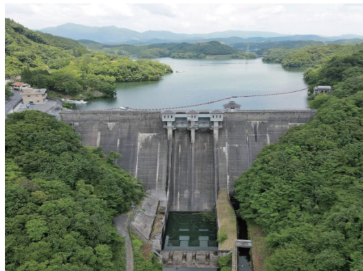
Figure 48 Hokuzan Dam Source: http://www.sa-tochi.jp/construction.html
