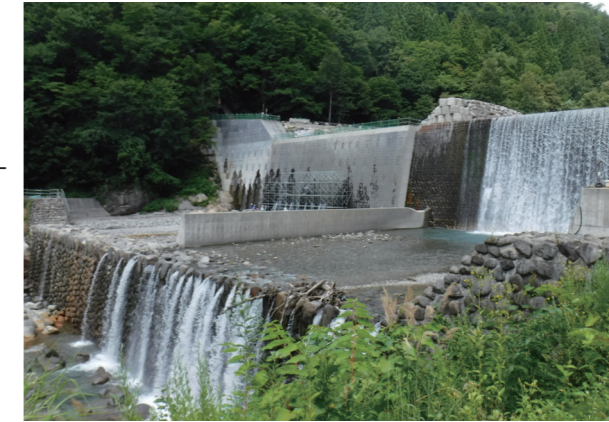
Figure 108 Sabo dam Source: https://www.hrr.mlit.go.jp/kanazawa/hakusansabo/09woman/fe16/fe16_0801.html
