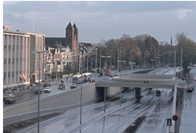
Figure 80 Catharijnesingel canal -Before- Source: https://worldlandscapearchitect.com/bringing-water-back-catharijnesingels-journey-back-from-highway-to-canal/?v=1a13105b7e4e
