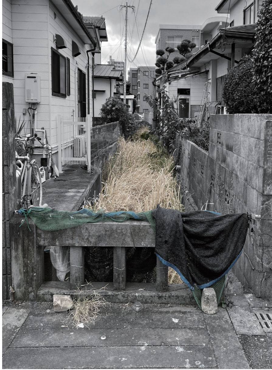
Figure 44 The overgrown canal in one of the residential area of Saga city
