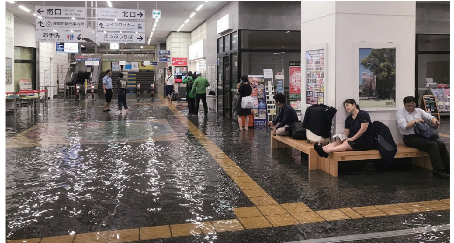
Figure 76 The flooded Saga station Source: https://www.nishinippon.co.jp/image/124146/
