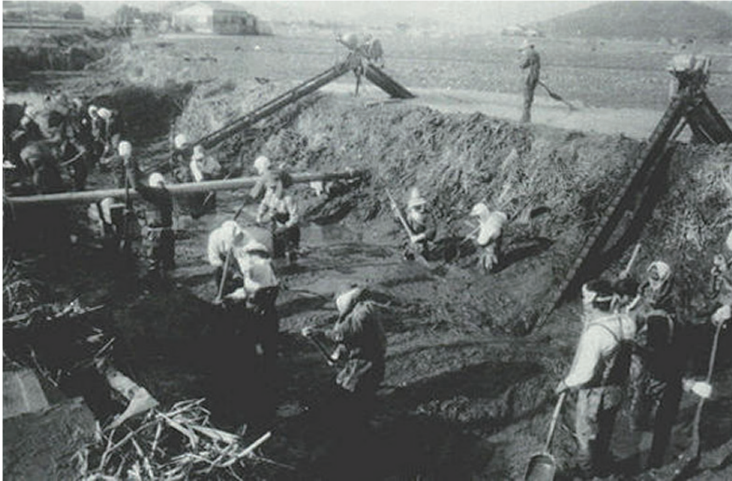
Figure 36 People dredging the canal (1955) Source: https://suido-ishizue.jp/daichi/part2/05/11.html
