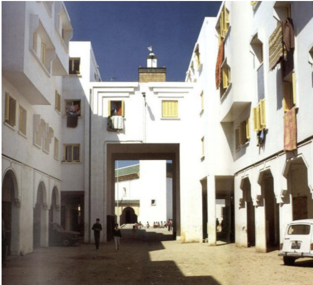
Fig. 30, Portal over a street in Dar Lamane Housing Project in Casablanca, Morocco (Maganga, 2025)
