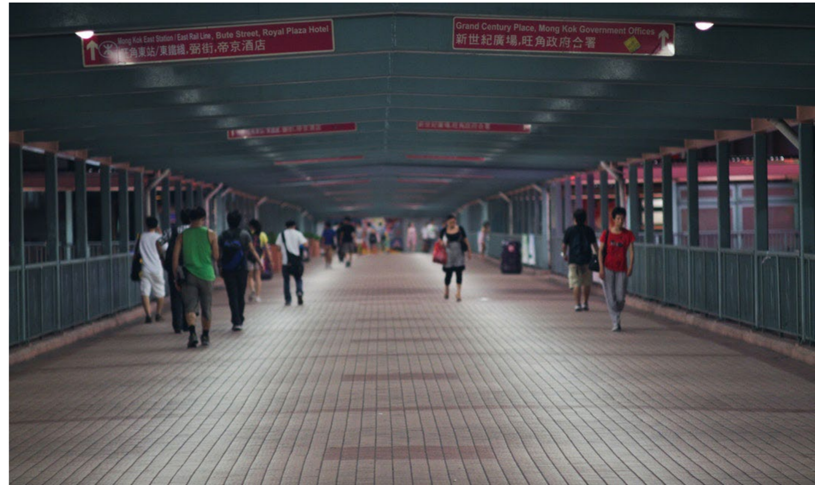
Mong Kok pedestrian footbridge Source from HKO1
