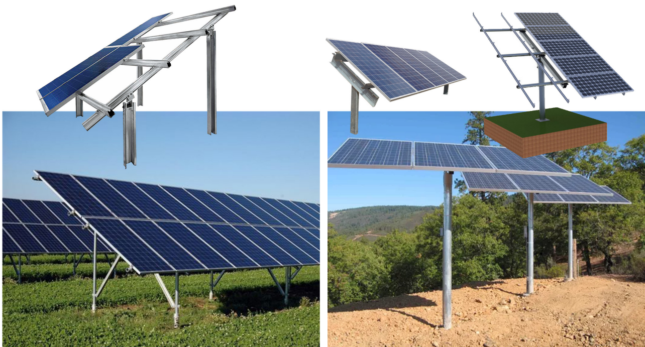
Figure 4.2, Ground mountings. Double posed mountings (left) and single posed mountings (right)
