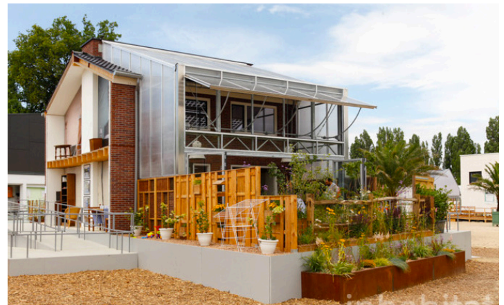
Picture 11: Pret a Loger, a second layer on top of a house [Inhabitat (2014)]
