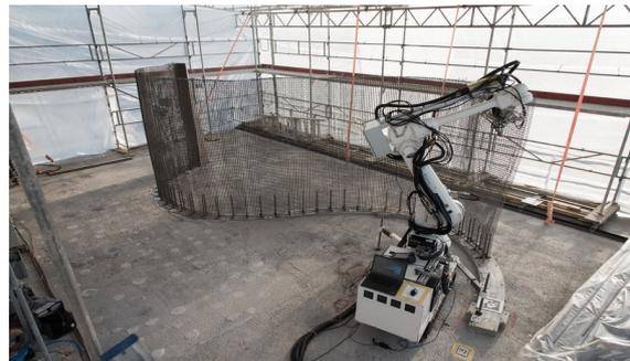
Figure 5.13: Mesh mould system at ETH Zürich [156]
