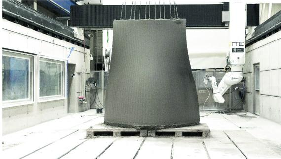
Figure 5.7: Reinforced curved wall using SC3DP [131]
