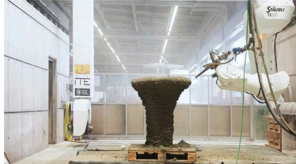
Figure 5.8: Cylinder with overhang using SC3DP [132]
