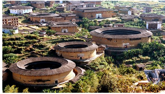
**Figure 3.9:** Tulou houses in Fujian, China built with rammed earth [33]
