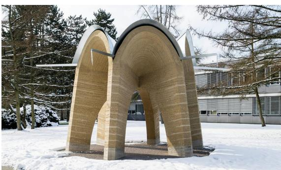
**Figure 1.8:** Prefabricated rammed earth pavilion
