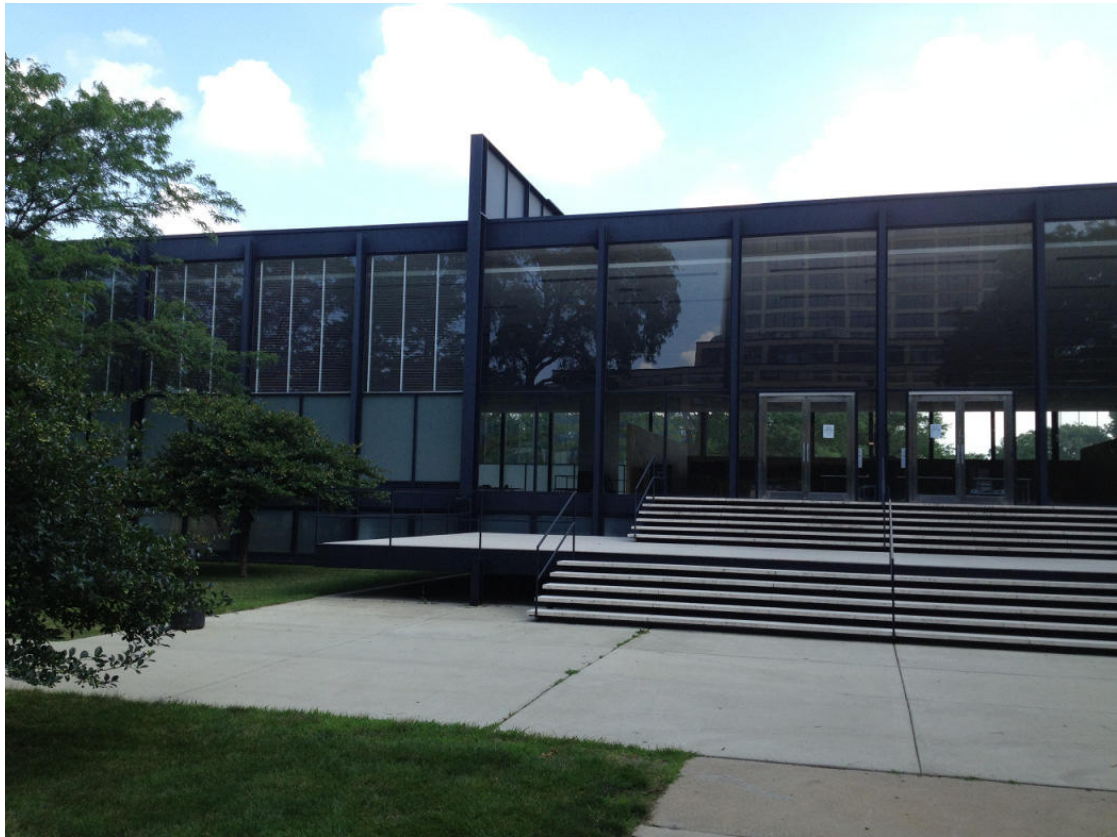
Fig. 10.7 Crown Hall, IIT (1950-1956), July 2013, photo by author. The building was closed at this point since, as IIT's own Michael Davis later told me, 'several leaks [had to be] fixed, windows replaced, woodwork cleaned, and so on.'
