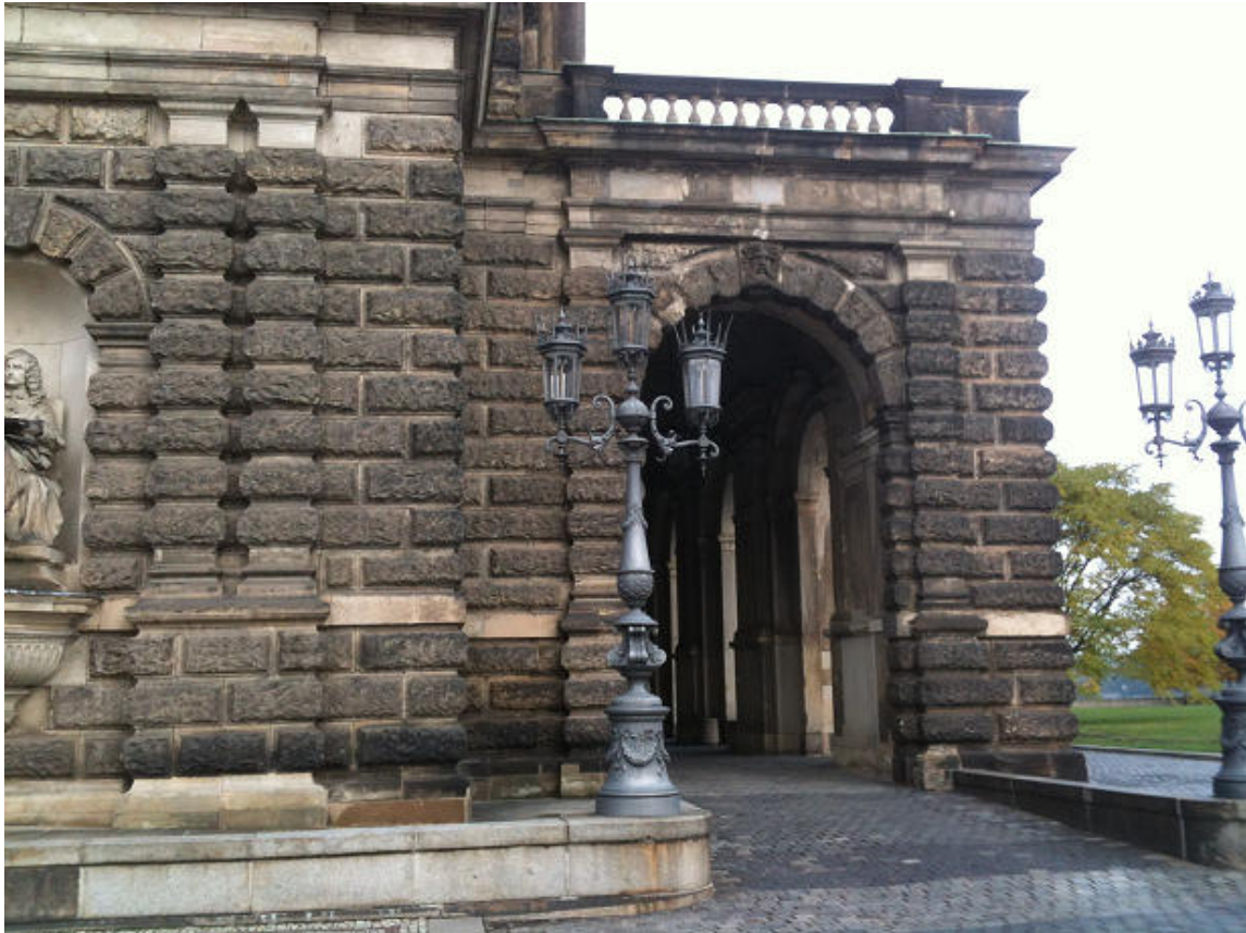
Fig 8.4b Semper’s Hoftheater , rustication detail. The drums on the columns are articulated individually.
