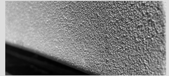
Figure 26 : Surface coating (Source: Parkitekt)
