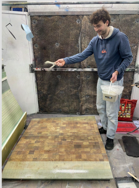
Figure 90: Applying antiskid granulate
