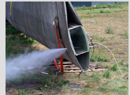
Figure 74: Rail guided water jet machine
