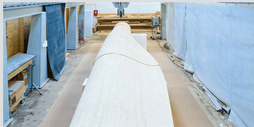
Figure 108: CNC mill shaping a wooden WTB (Voodin, 2024) (Source: balticwind.EU)
