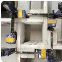
pouring the mixture into the form
