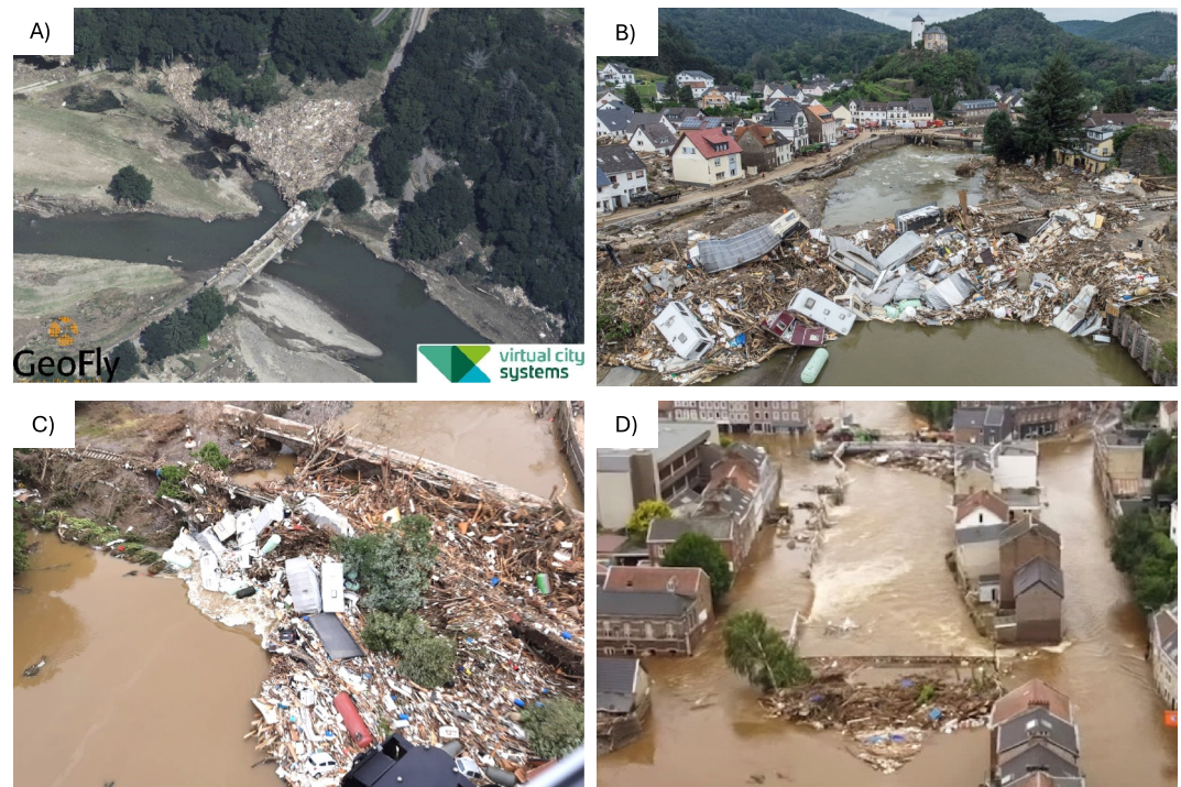
Figure 5. Examples of clogged bridges in the database. (a) Pützfeld, Germany (bridge ID 63 in the database by Erpicum, Poppema, Burghardt, Benet, Klopries, et al. (2024)). Photo based on an aerial survey after the flood event by GeoFly GmbH and provided by Virtual City Systems. (b) Kreuzberg, Germany (bridge ID 62, after the flood). Source: Baumert (2024). (c) Altenahr, Germany (bridge ID 55 and 56, after the flood). Photo by Polizei Thüringen (2021). (d) Pepinster, Belgium (foreground: bridge ID 59; background: bridge ID 60, during the flood) Credit: Vedia. The flow direction is from left to right and foreground to background.
