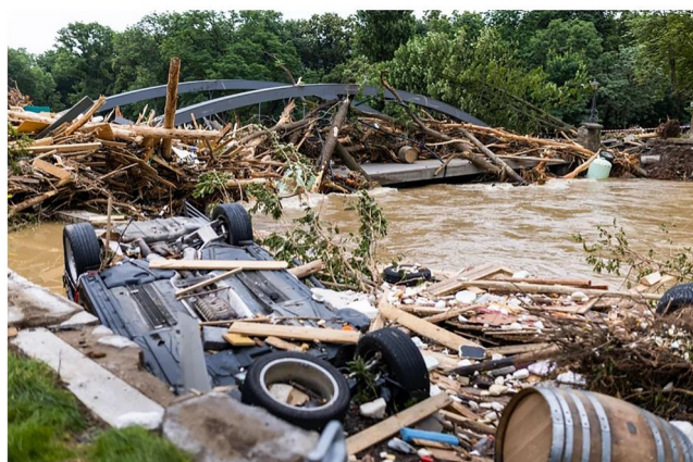
Figure 1. A debris accumulation in Bad Neuenahr-Ahrweiler, Germany (bridge 16 in the database by Erpicum, Poppema, Burghardt, Benet, Klopries, et al. (2024)). Trees, vehicles, tanks and other objects are present in front and on top of the bridge, with debris interlocking with the bridge superstructure. Photo by Philipp von Ditzfurth (Jannaschk, 2021).
