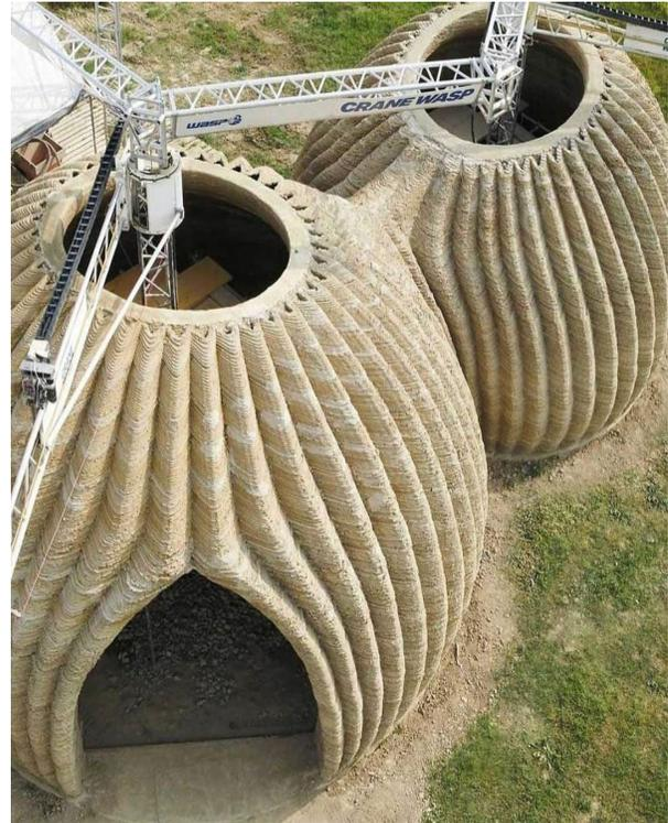
*Figure 3: Prototype printing of the Tecla house. Source: <https://parametrichouse.com/tecla/>*
