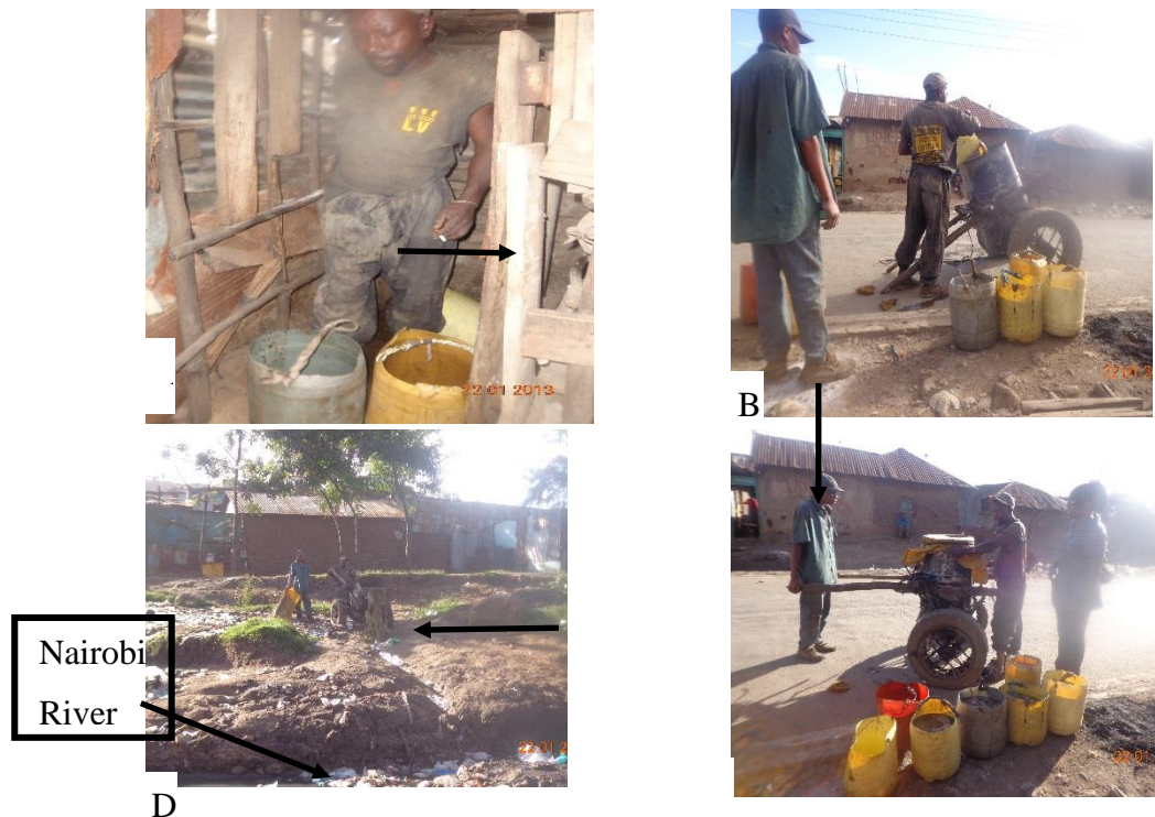
Figure 2.8: Pictures illustrating faecal sludge management activities A) Latrine desludging, B) and C) Preparation for transportation, D) Dumping in Nairobi river
