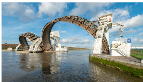
Figure 1.3: Weir complex in Driel [13]
