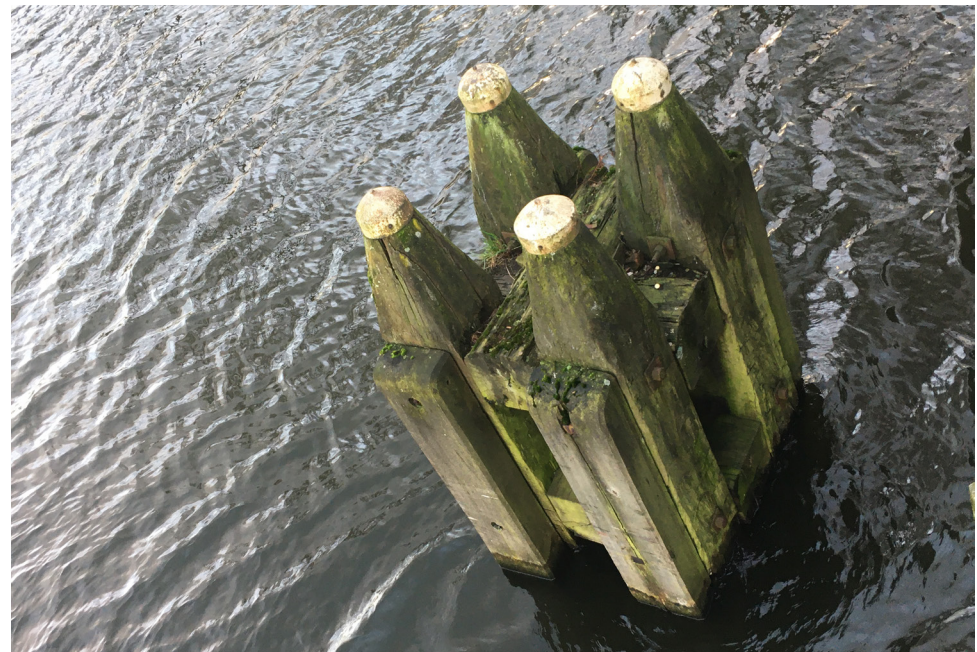
Used mooring poles: normally 400 x 400 mm with a length of 15 meters
