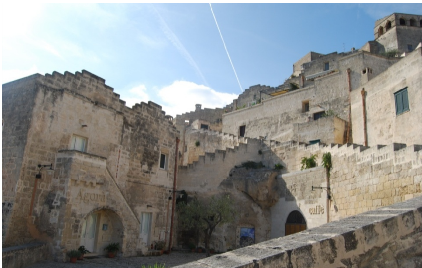
The settlement of Sassi, in Matera, Italy showing the intensive use of thermal mass to reach comfort level throughout the hot and cold seasons. Source: Author
