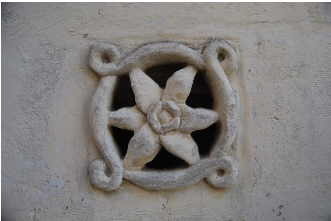
Embedded Ventilation functions in the local limestone of Matera, named 'Tufo', Sassi di Matera, Italy
