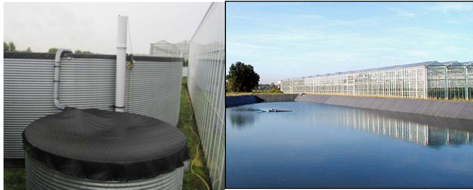
Figure 3.7: Greenhouse storage facilities: silo (left) and basin (right)
